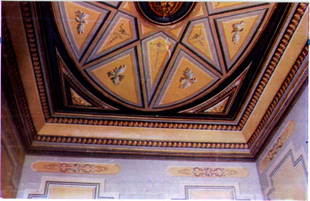
The ceiling ornaments before restoration
