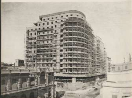
View of the building in progress.
