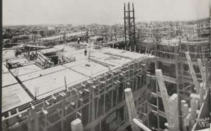
View of the site at the end of construction
