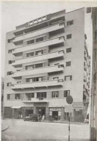
Appartement KAHIL 17, Avenue 1700
