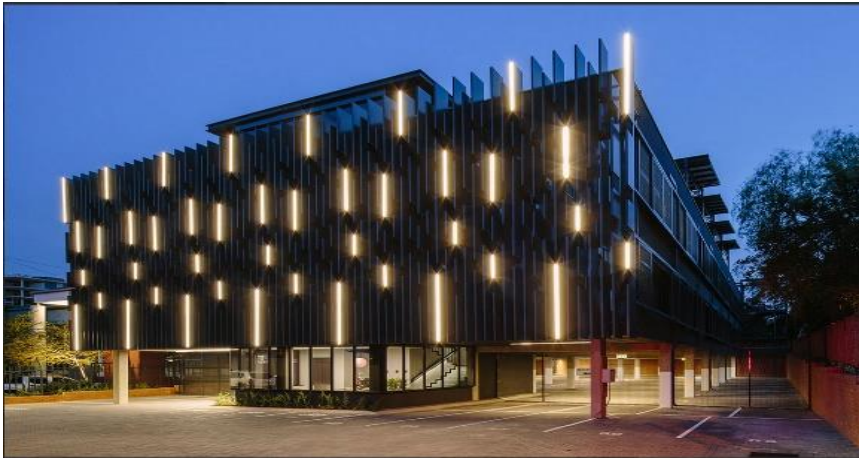
Fig.3.19 : 78 Corlett Drive building 54
