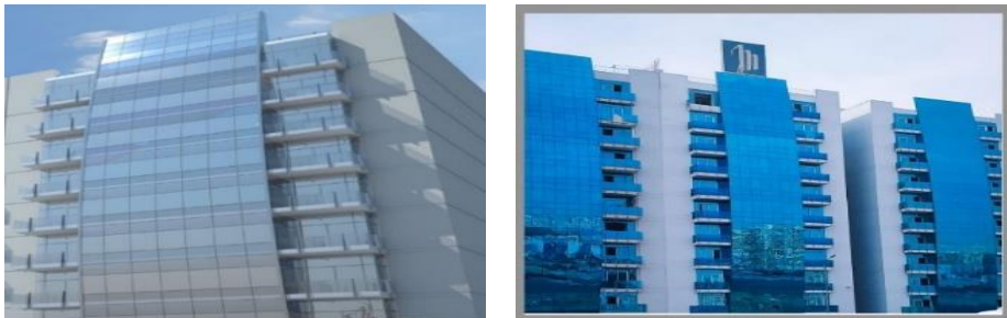
Fig.4.7: The façade of the office building
