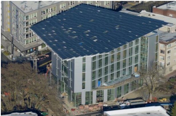
Fig.3.4: Solar Panels on the Bullitt center 17
