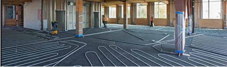
Fig.3.7: Tubing for in-floor radiant heating or cooling 25 .
