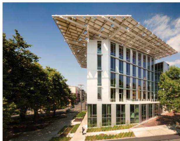
Fig. 5: The Bullitt Center building[42]
