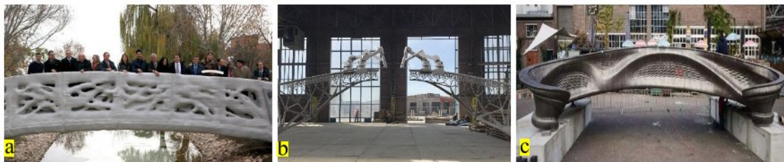
Fig. (2) (a) 3D printed bridge with the D-Shape technology. The first structure of this type in the world [7] , (b) 3D-printed steel bridge in the heart of Amsterdam 3D-printed steel bridge in the heart of Amsterdam, (c) the first 3D-printed steel bridge. In 2015, Dutch 3D printing company MX3D [8] .
