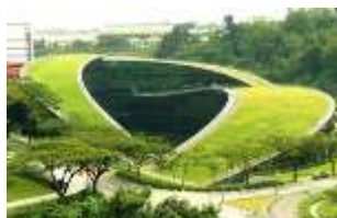
Fig.10. The green roof of the Faculty of Fine Arts in Singapore( https://al )
