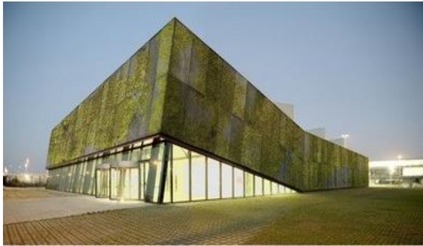
Figure 7. Biological concrete to create green facades for the Aviation Cultural Center
