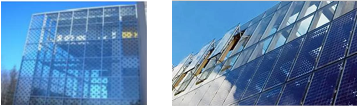
Figure 10. Shows glass equipped with solar cells
