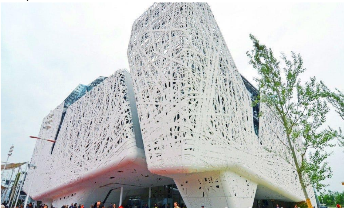
Figure 6. Shows the use of pollution-reducing cement in the Palazzo-Italia building with a bio-green, air-purifying atmosphere
