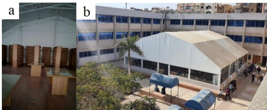
Figure 20 (a) the location of the library building with a trussable structure in the middle of the campus and the places of the windows, (b) the shelves area inside the library and the lack of natural lighting to reach the area and no artificial lighting.
