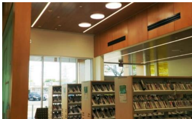
Figure 17 Solatube at South Whittier Public Library.
