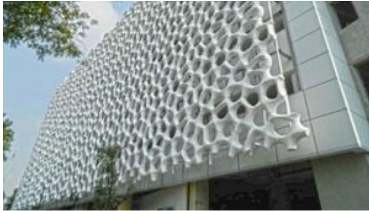
figure (3) illustrates the hospital façade of (Torre de especialidades)
