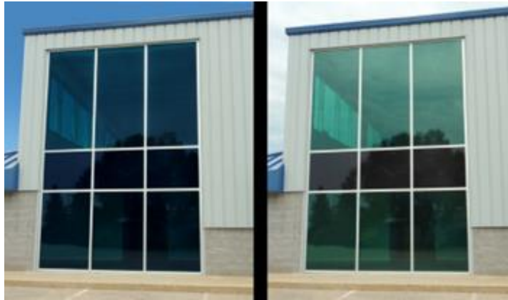
Fig.8 The effect of lighting on the color and transparency of glass used with photochromic technology.
