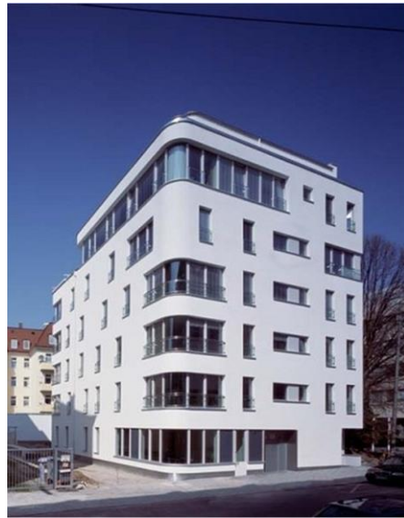
Fig.7 The Seitzstraße apartments with Vacuum Insulated Panels.(Arif,2020)
