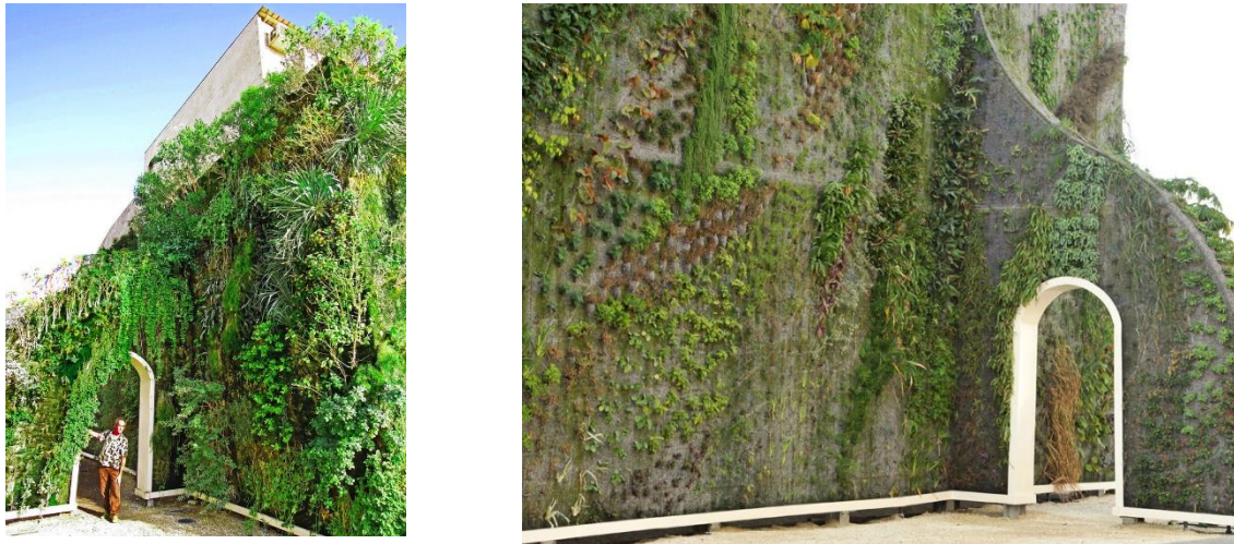
Figure (1) The vertical garden at the Sheikh Ibrahim bin Mohammed Al Khalifa Center
