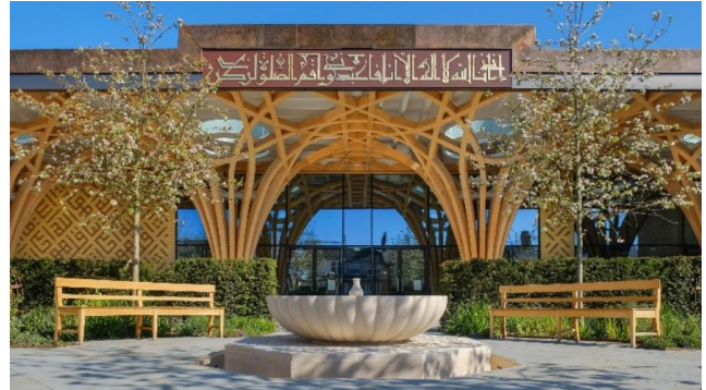
Figure 7 Tree-like pillars form the structure of the Cambridge Central Mosque. Above: the design was based on the idea of a "calm oasis". Source: https://www.dezeen.com/2021/01/20/cambridge-central-mosque-marks-barfield-architects/
