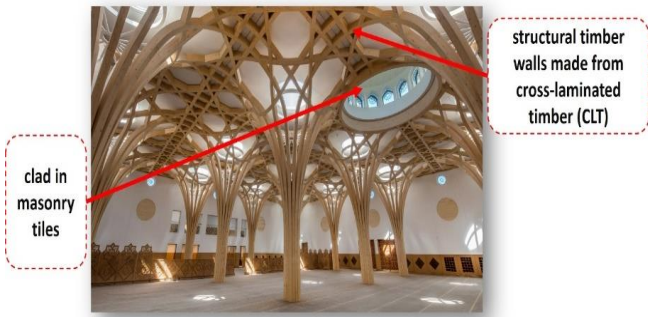
Figure 12 Prayer Hall structure features digitally fabricated tree timber columns supporting the roof structure. Source: “ https://www.dezeen.com/2021/01/20/cambridge-central-mosque-marks-barfield-architects .”
