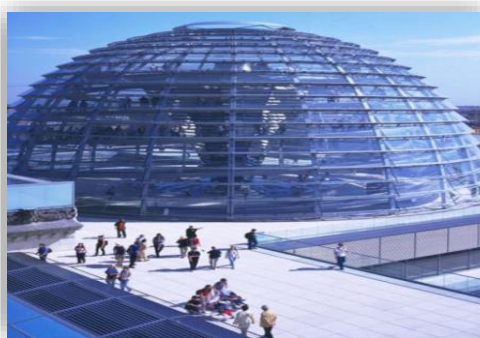
Figure (17) shows an external image of the glass dome connected between the internal and external environment by means of the advanced building technology
