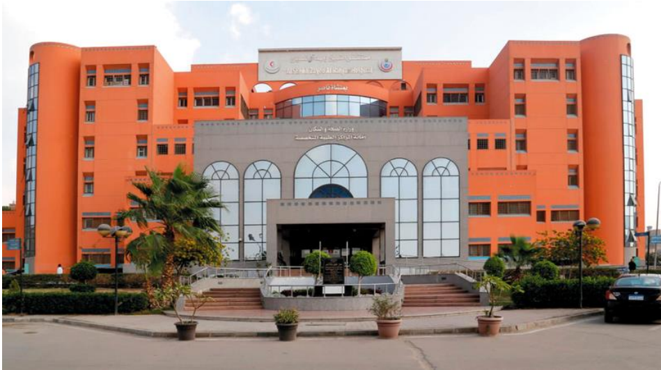
Figure 4- 35: El-Sheikh Zayed Al Nahyan Hospital
