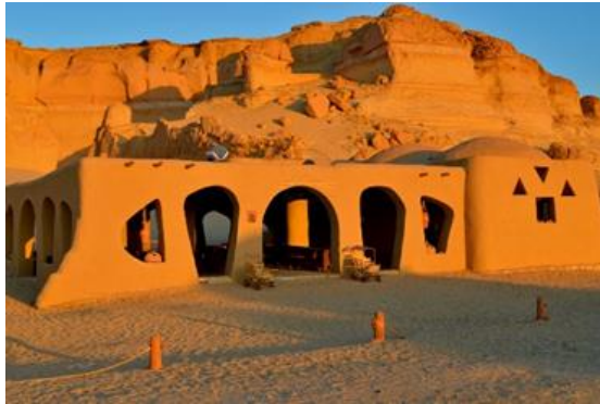
Figure (46): The visiting facilities in the Wadi AL-Hitan protectorate located in Fayoum are built from adobe bricks with load-bearing walls, vaults, and domes produced from locally desert clay. Eco-Architecture is the project's designer.
