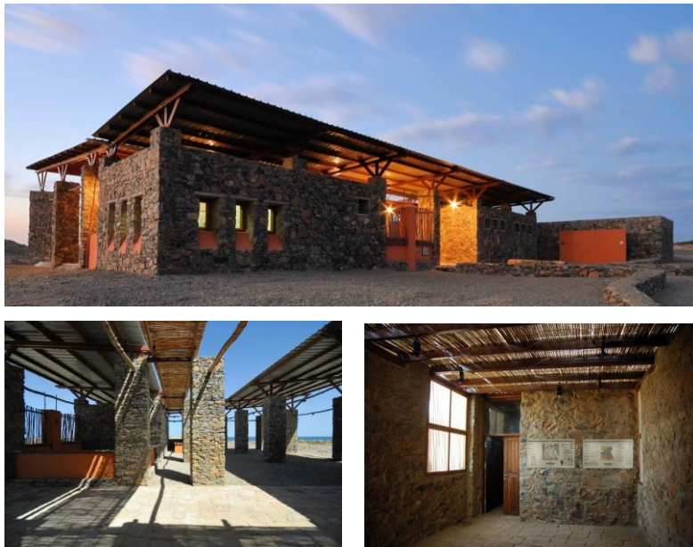
Figure (47): Visitors Center in Marsa Alam's Wadi Al-Gemal protectorate, built with local stone bearing walls and corrugated sheet roofs. Project architects: EECA
