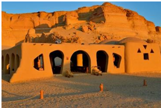
Figure (36): The visiting facilities in the Wadi AL-Hitan protectorate located in Fayoum are built from adobe bricks with load-bearing walls, vaults, and domes produced from locally desert clay. Eco-Architecture is the project's designer.
