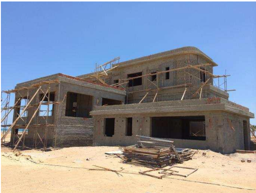
Figure (54): El Gouna single-family home under construction.
