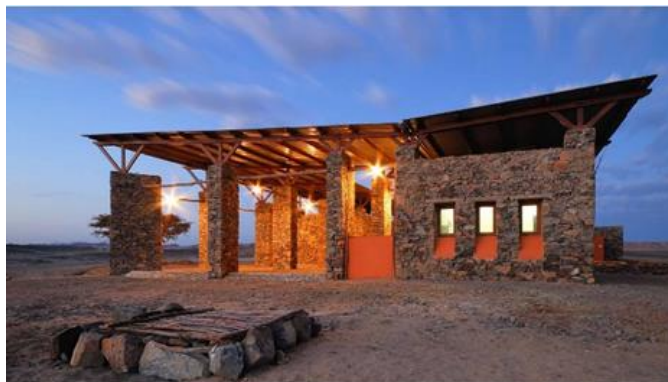
Figure (37): Visitors Center in Marsa Alam's Wadi Al-Gemal protectorate, built with local stone bearing walls and corrugated sheet roofs. Project architects: EECA
