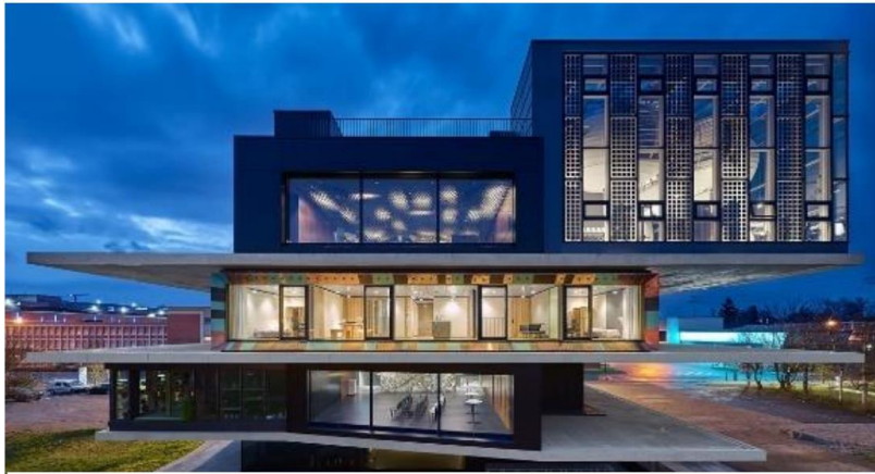
Figure (18): The Urban Mining and Recycling (UMAR) Experimental Unit is built mainly by materials which is recyclable, reusable, and compostable. (Architects: Werner Sobek, Dirk E. Hebel & Felix Heisel, Photo: Zooey Braun)
