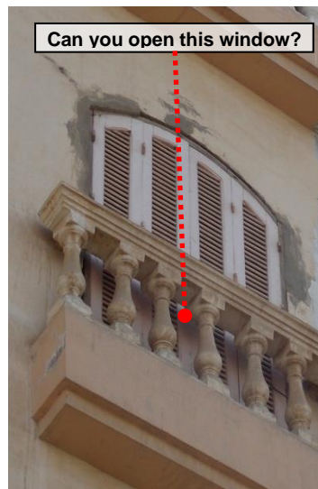
Fig. 13: wrong design for window and elevation (Al-Tawansy,2013)
