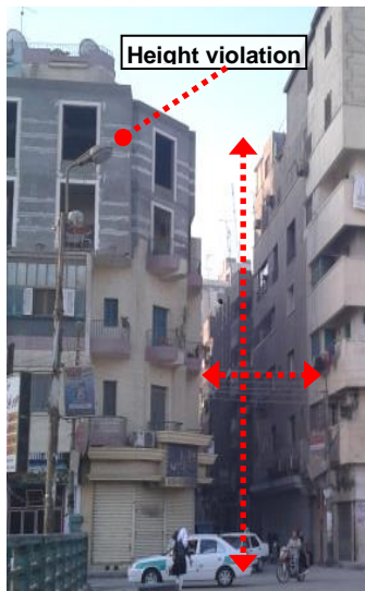
Fig. 12: Building has two additional unlicensed floors (Al-Tawansy,2013)
