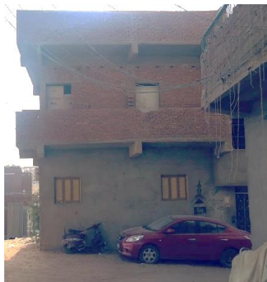
Reinforced concrete and burned clay bricks in a new house, Khargh
