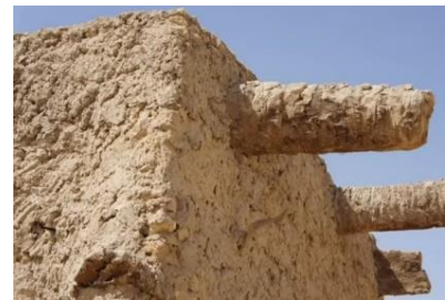
Karsheef walls and palm trunks for ceiling, Shally, Siwa
