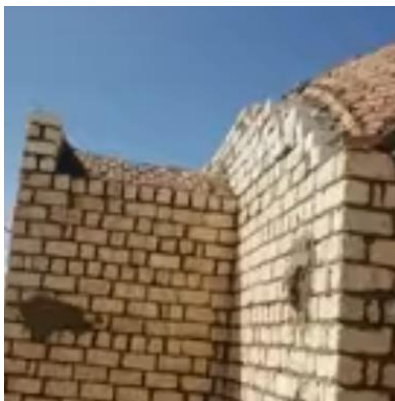
Limestone bearing walls and brick vaults in a farmhouse, Bahariya
