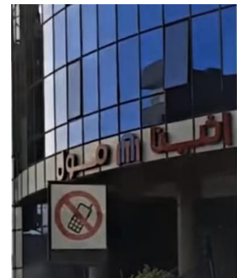
Glass Curtain walls, Athena Mall, Dakhla
