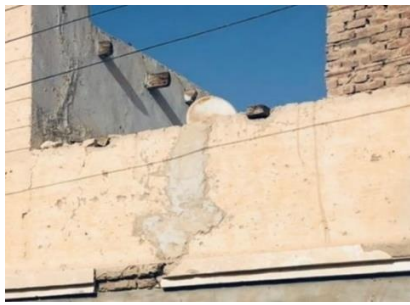
Cement plaster on mud bricks, Kharga, Author.
