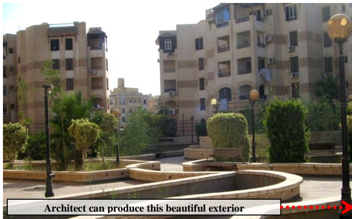
Fig. 10: A luxury housing project reflects that the architect focus of interest is aesthetics, ignoring the technical aspects, Author.
