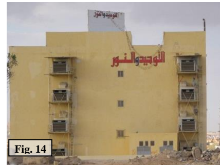
Fig. 12→14: Architect unawareness of electromechanical special needs caused these ugly malls exteriors, Author
