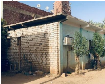
B- Bearing walls of stone & reinforced concrete ceiling
