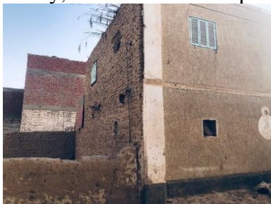
A- Bearing walls of mud bricks & palm trunks & Leaf
