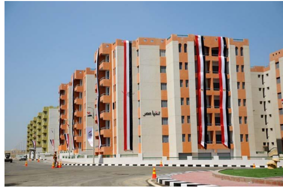
Fig (12): Dorrat Alwady Governorate recent Housing Project in 2022 at Al khargah (Qasr), Author , 2022.
