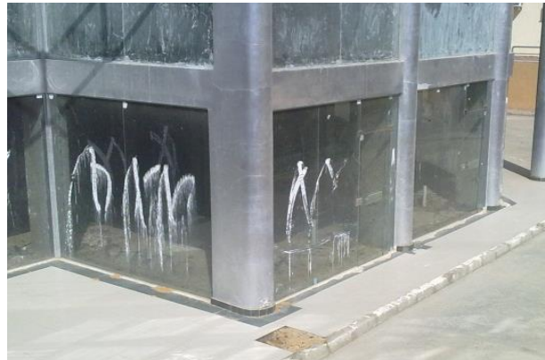
Fig. 9: Mall Glass Façade. Source: Author.
