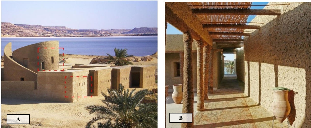
Fig. 18: Ecolodge tourist hotel at Siwa by Laetitia Delubac and Christian Félix architects, Paris, France, Pic. Source: Web Network.
