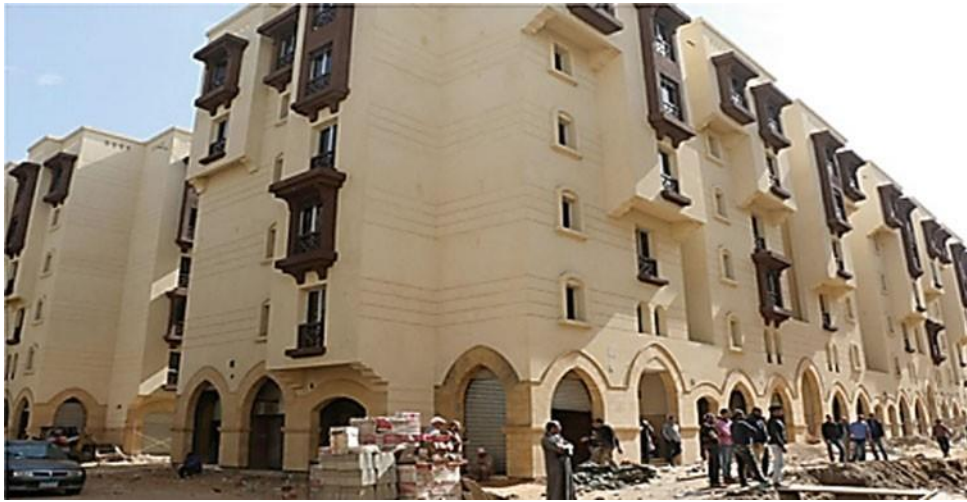
Fig. 4 Al-Sayeda Zeinab Kindergarten (Tal Al- Aqarib Project)
