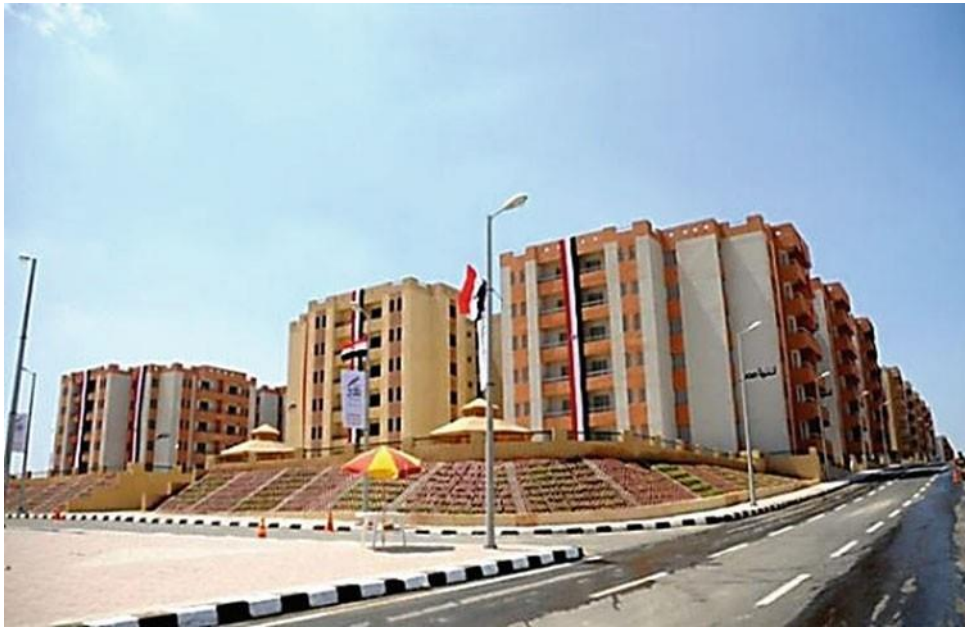
Fig. 7 Residential buildings Al Asmarat Project in Mokattam
