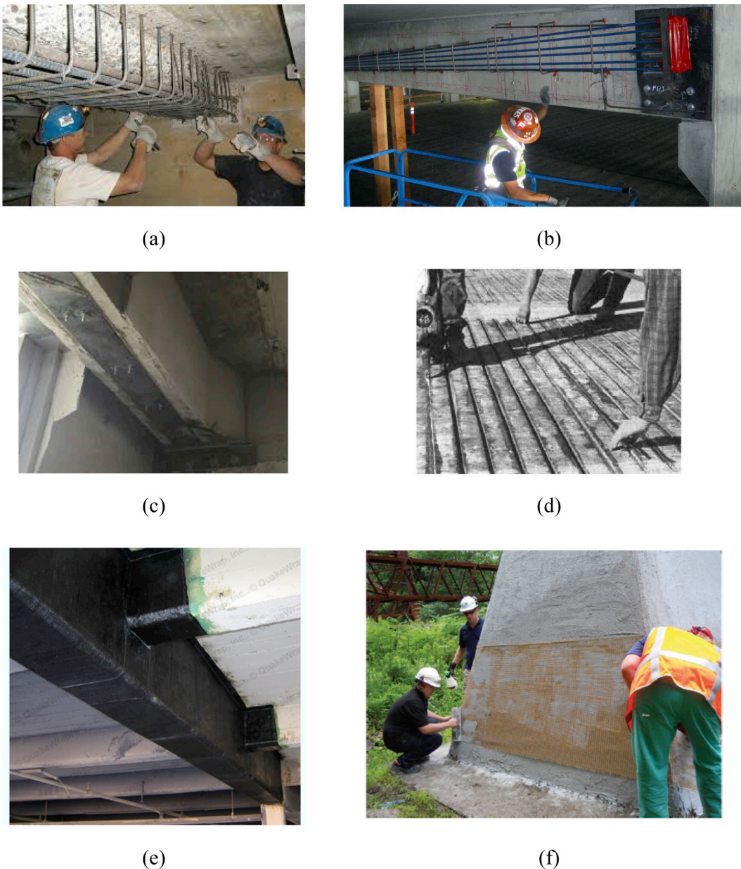
Fig. 1. Examples of strengthening techniques of concrete structures: (a) Section enlargement [19]; (b) External post-tensioning [21]; (c) Steel plate bonding [22]; (d) NSM strengthening [24]; (e) FRP strengthening [26]; (f) TRM strengthening [31].
