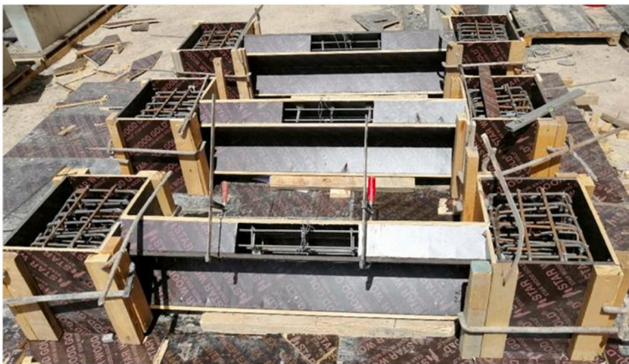
Fig. 3. Steel cages of specimens in the formwork ready for concrete casting.
