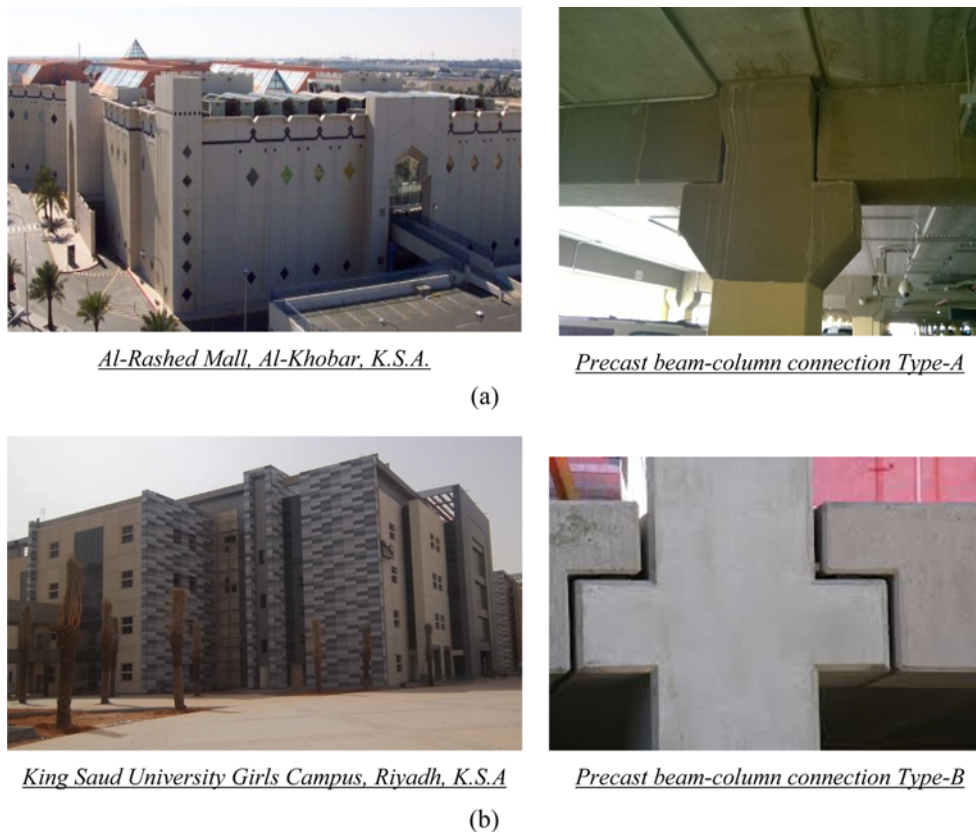
Fig. 1. Examples of Typical Beam-column Connections in Precast Buildings in Saudi Arabia: (a) Precast Type-A Beam-column Connection, (b) Precast Type-B Beam-column Connection
