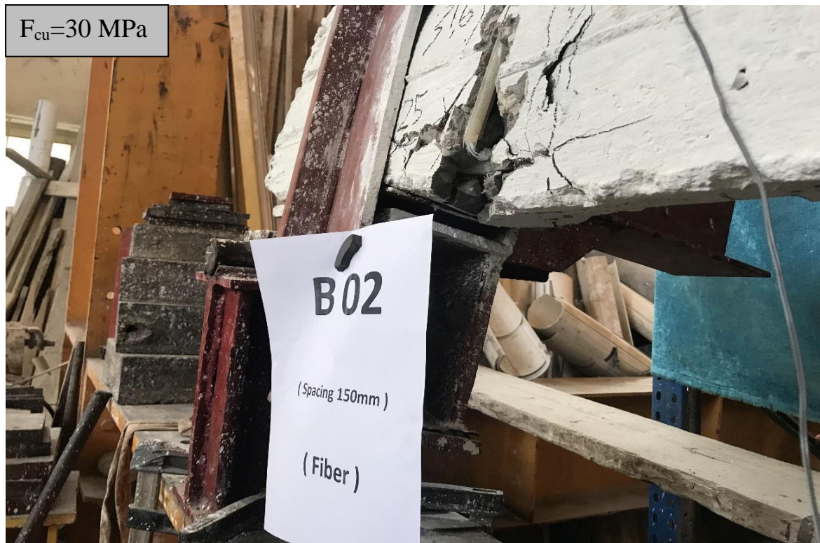
Figure (5-26-a) Rupture in Stirrups for Specimen B2.
