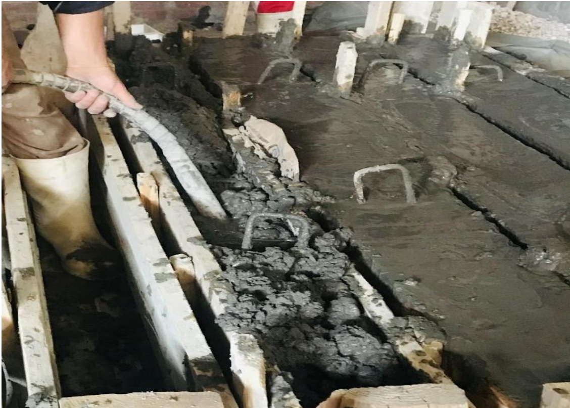
Figure (3-9): Compaction of Concrete
