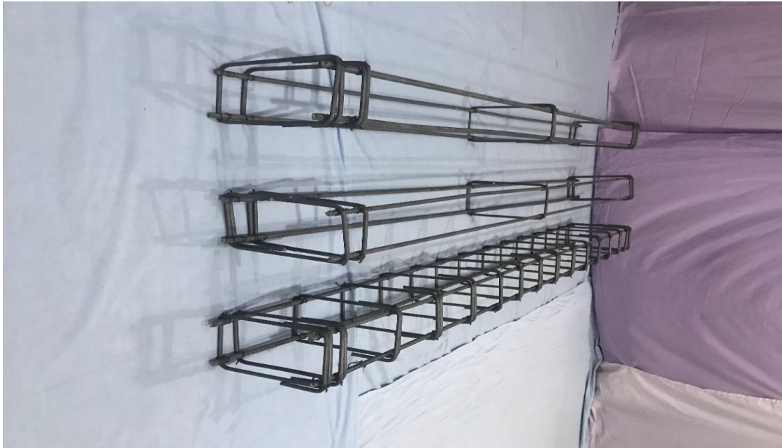
Figure (3-7): Steel Reinforcement Details of Beams.
