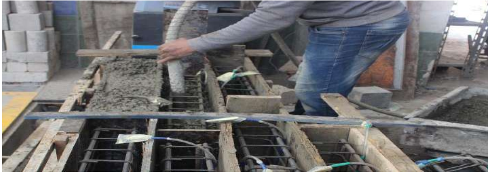
Figure (3-17): A mechanical vibrator to ensure full compaction of concrete.
