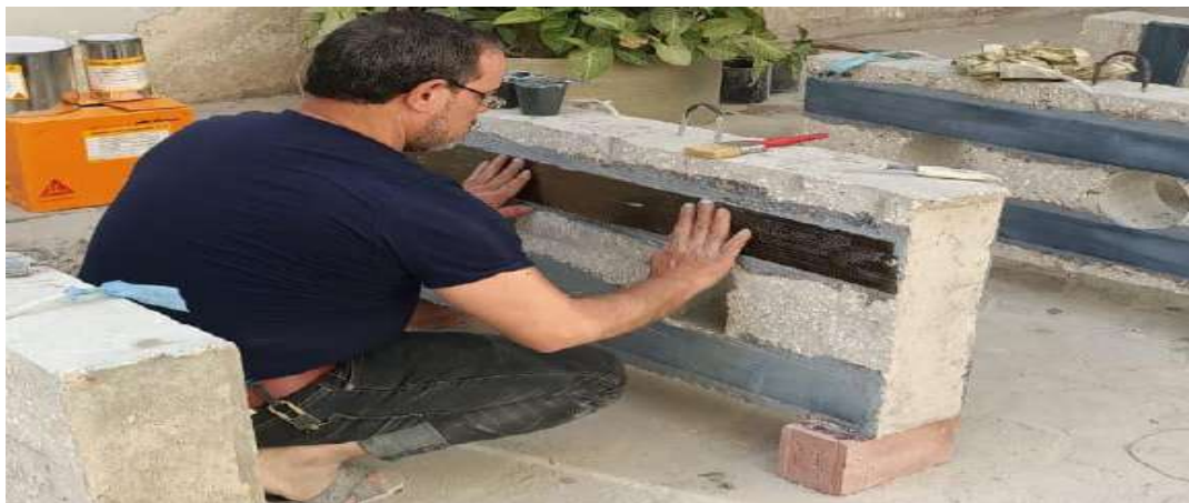
Figure (3-23): The composite fabric placed on top of epoxy resin coating
