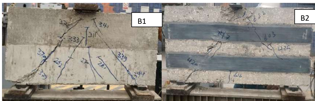
Figure (5-1): Crack pattern for deep beams without openings
