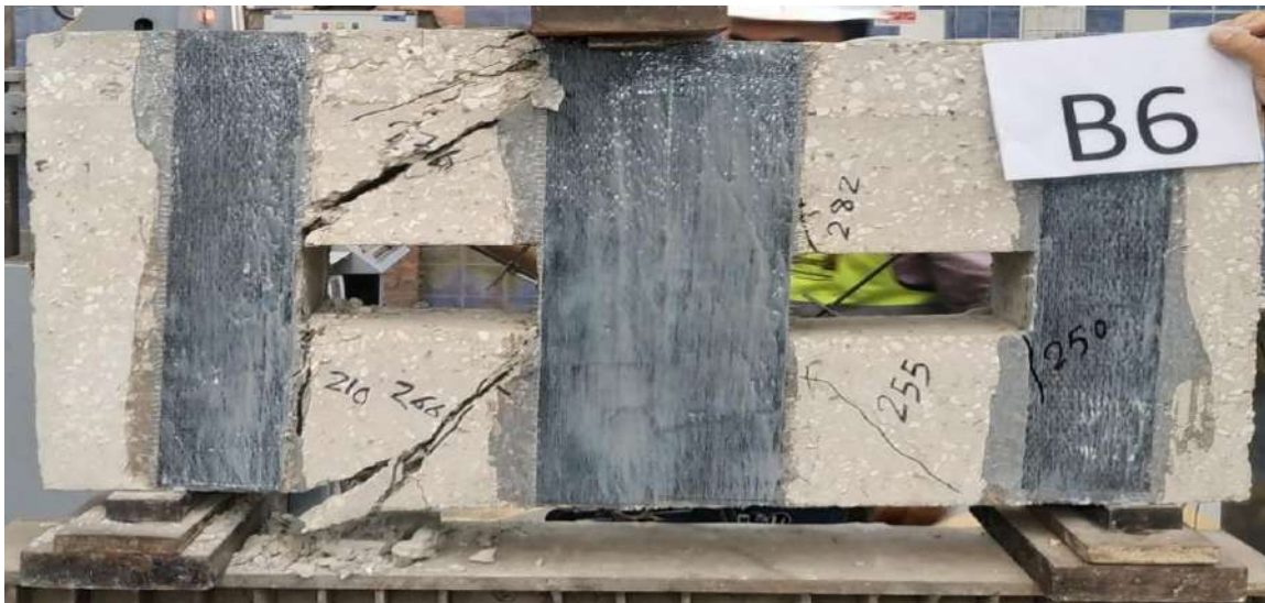
Figure (4-6): Crack pattern of the beam (B6) at failure
