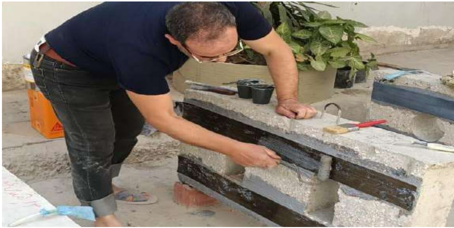
Figure (3-24): The second layer of the epoxy resin
