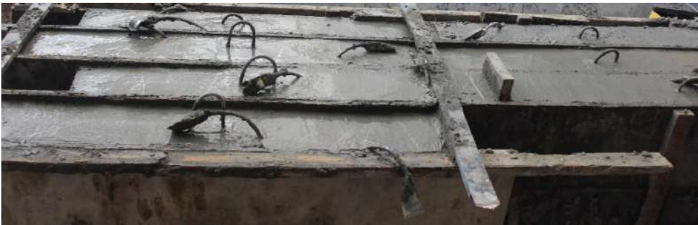
Figure (3-18): The beams after casting and leveling the surface.
