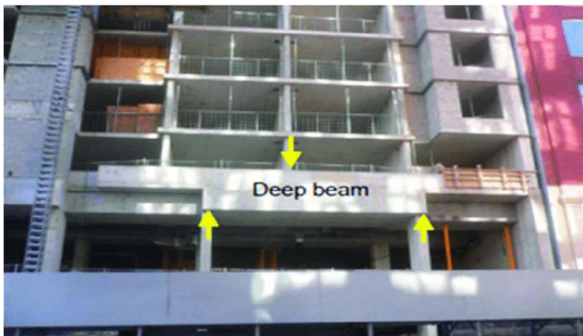
Figure (2-7): Applications of deep beams
