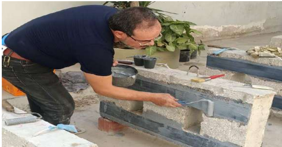
Figure (3-25): The resin was squeezed through the roving of the fabric
