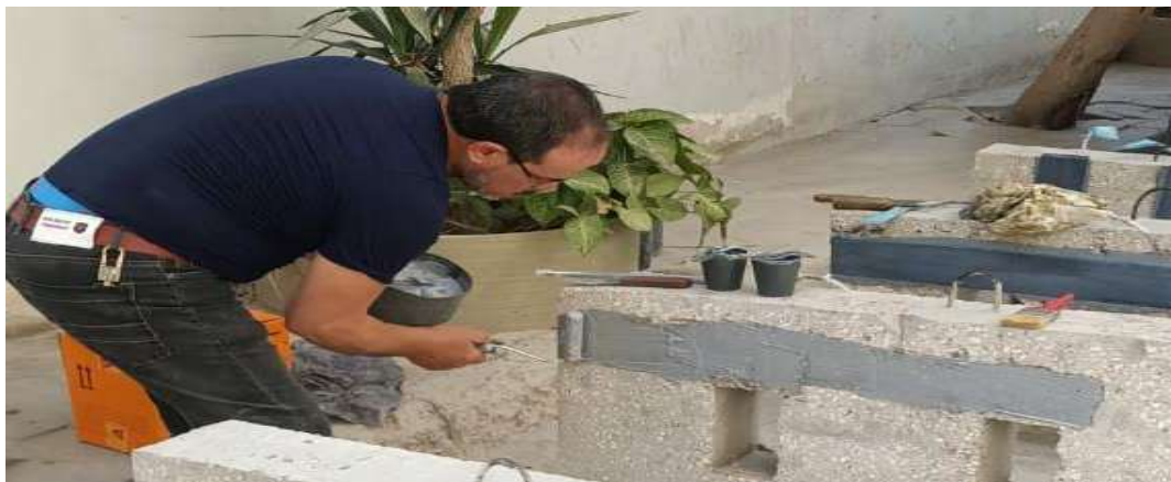
Figure (3-22): Epoxy resin applied to the concrete surface
