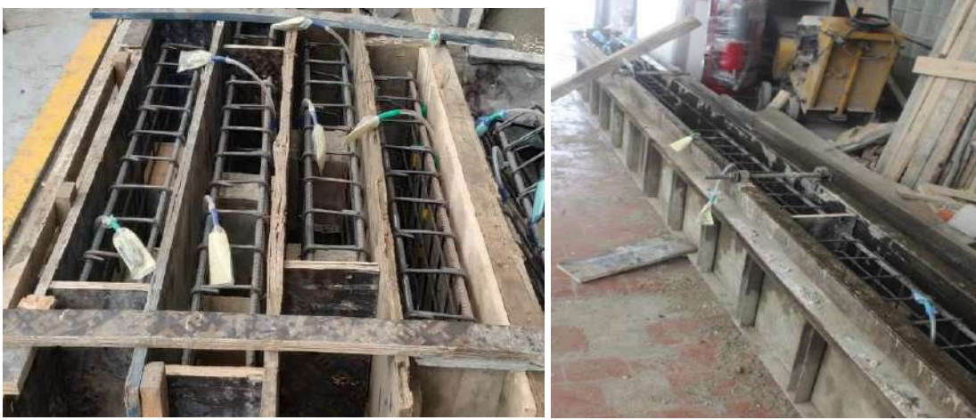
Figure (3-14) Wooden and steel form used in casting the specimen
