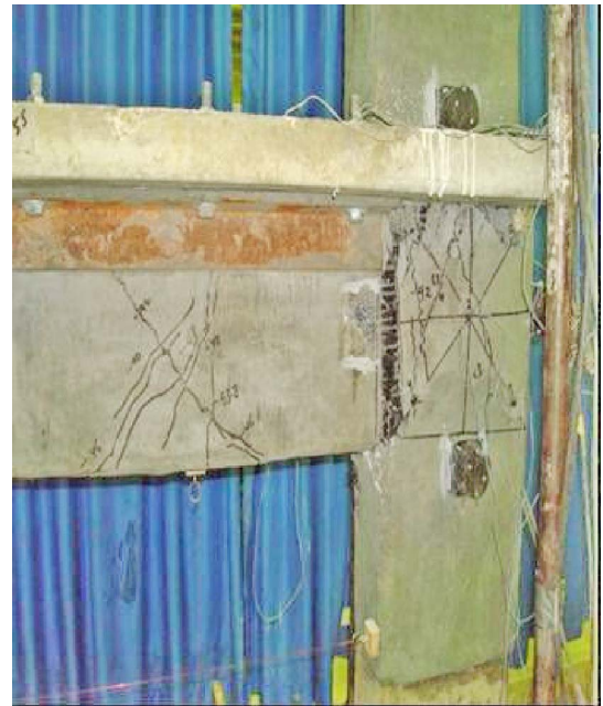
Fig. 18. Failure pattern of TRM-strengthened specimen (image by the authors)
