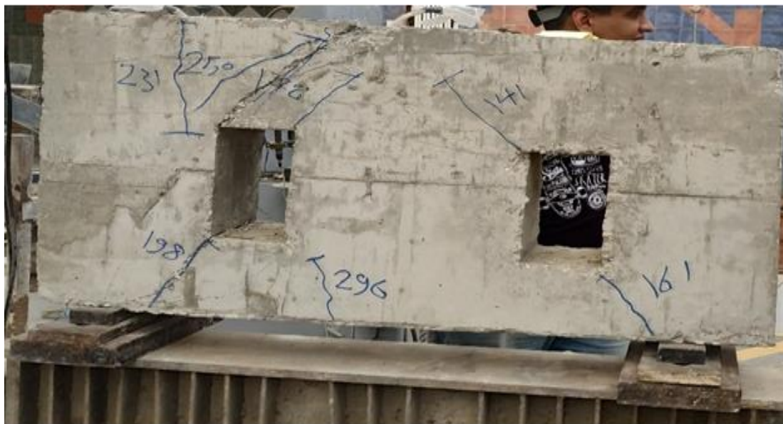
Figure (6): crack patten of control deep beam (NS-VRO)
