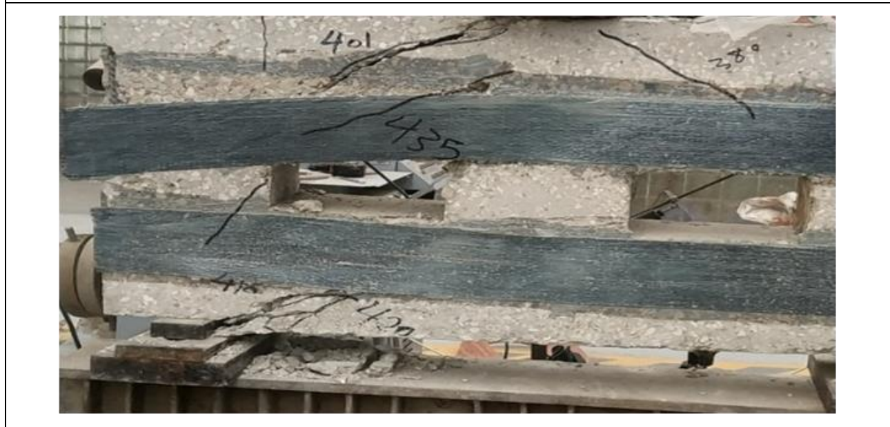
Figure (8): crack patten of deep beam with horizontal openings strengthened with horizontal BFRP (HS-HRO)
