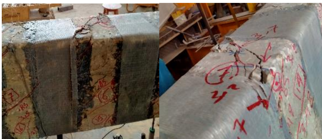
Figure 15 : Failure mode of beam G3 wrapped with vertical glass strips.
