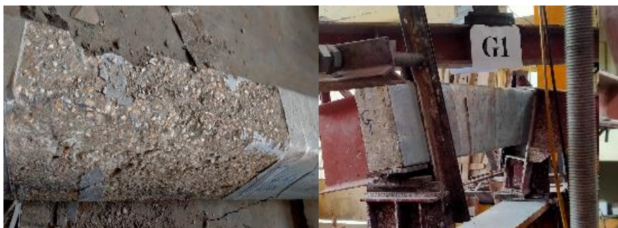
Figure 12 : Cracks Pattern in G1 after removal of FRP .
