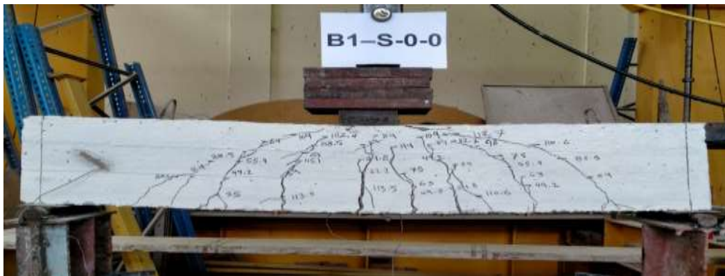
Figure (2): Cracks for Beam (S-0-0) at Failure
