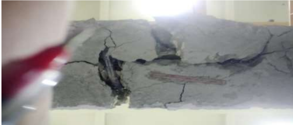
Figure (5): Typical Splitting Failure of Concrete in the Tension Zone
