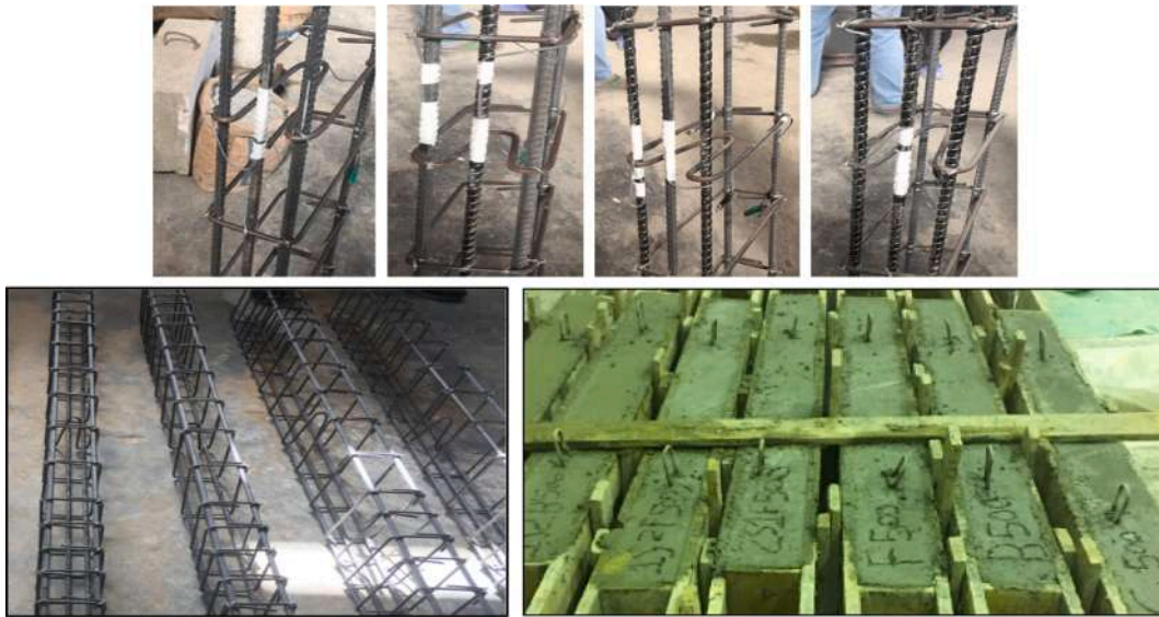
Fig. 4. Details of Reinforcement and Wooden Forms.
