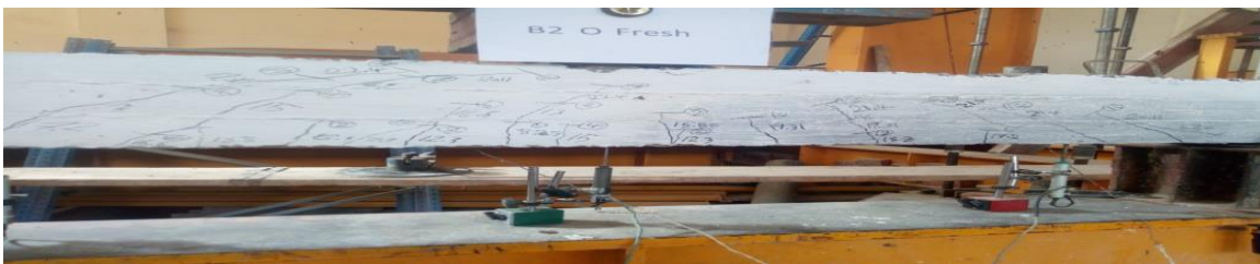
Fig.(14).Cracking Pattern for Beam (B2OF).
