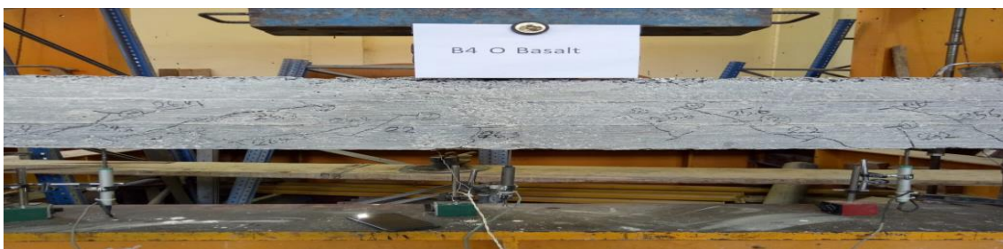
Fig.(15).Cracking Pattern for Beam (B4OB).
