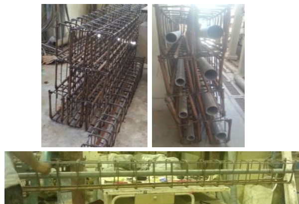
Fig. 12 Reinforcing Cages and Holding PVC Pipes
