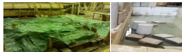
Fig. 15 Curing of Cubes, Cylinder and Beam Specimens
