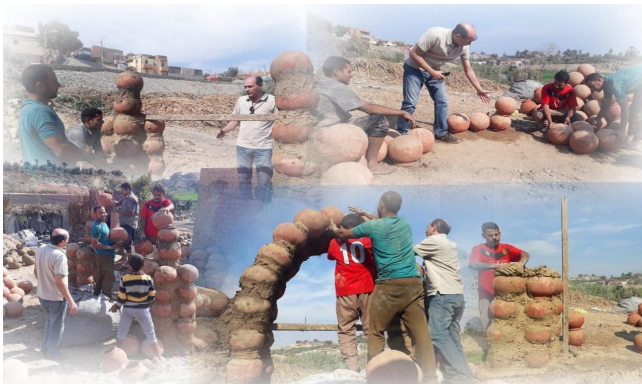
Figure 7. The Construction Experimentation Using the Pottery Unit, El-Setouhy, 2021.
