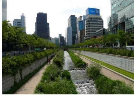
Figure 16: Natural Stones in Areas of slower or still water to support biodiversity and aquatic life.
