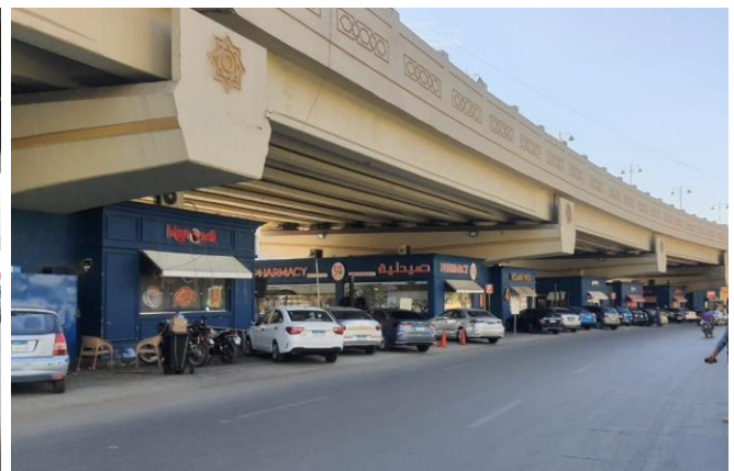
Figure 2 The current situation in Egypt below the elevated road El-Etahdya in Masr El-Gadida. source: researcher
