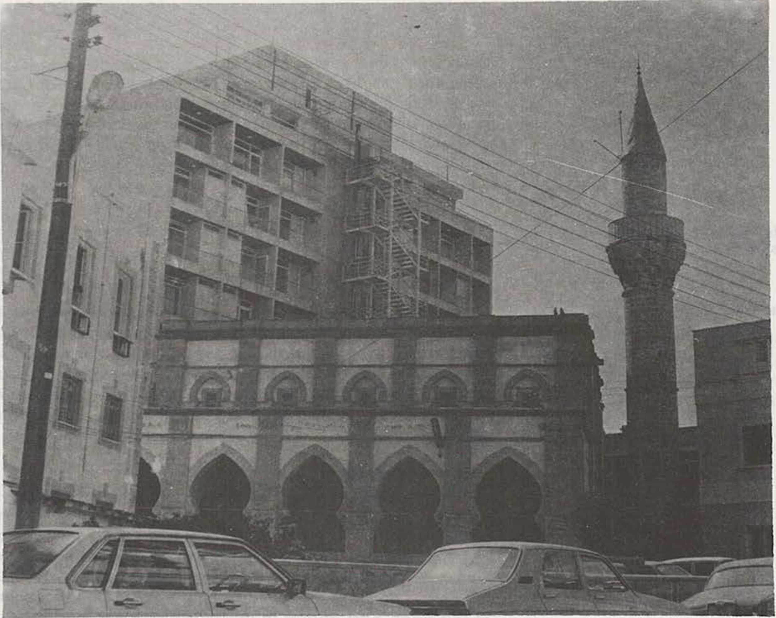
- Sarayonu mosque. The adjacent hotel has ruined the architectural and historic characteristic style.
