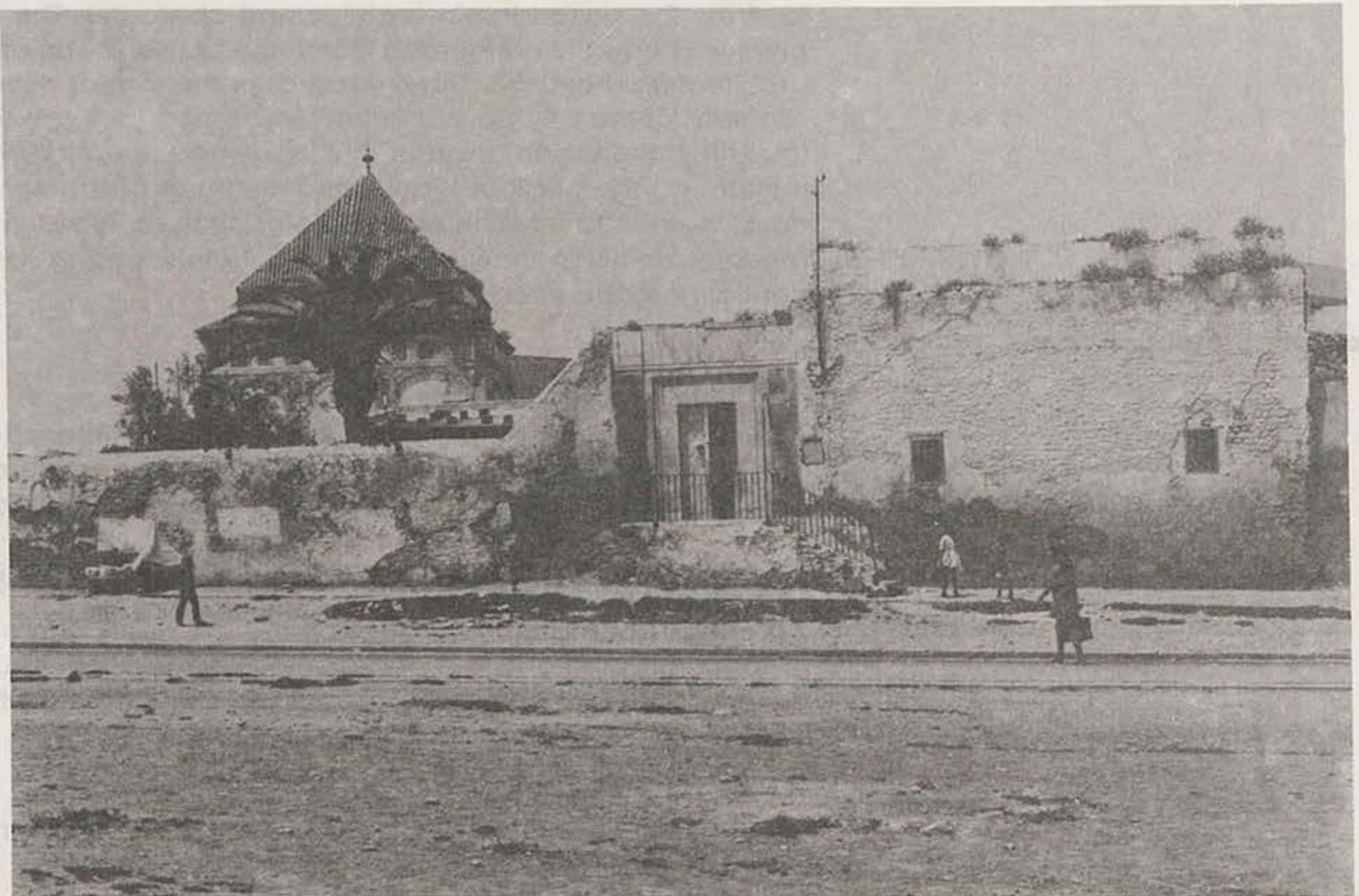
- Zawia of Sidi Qasem before restoration - Old City of Tunis
