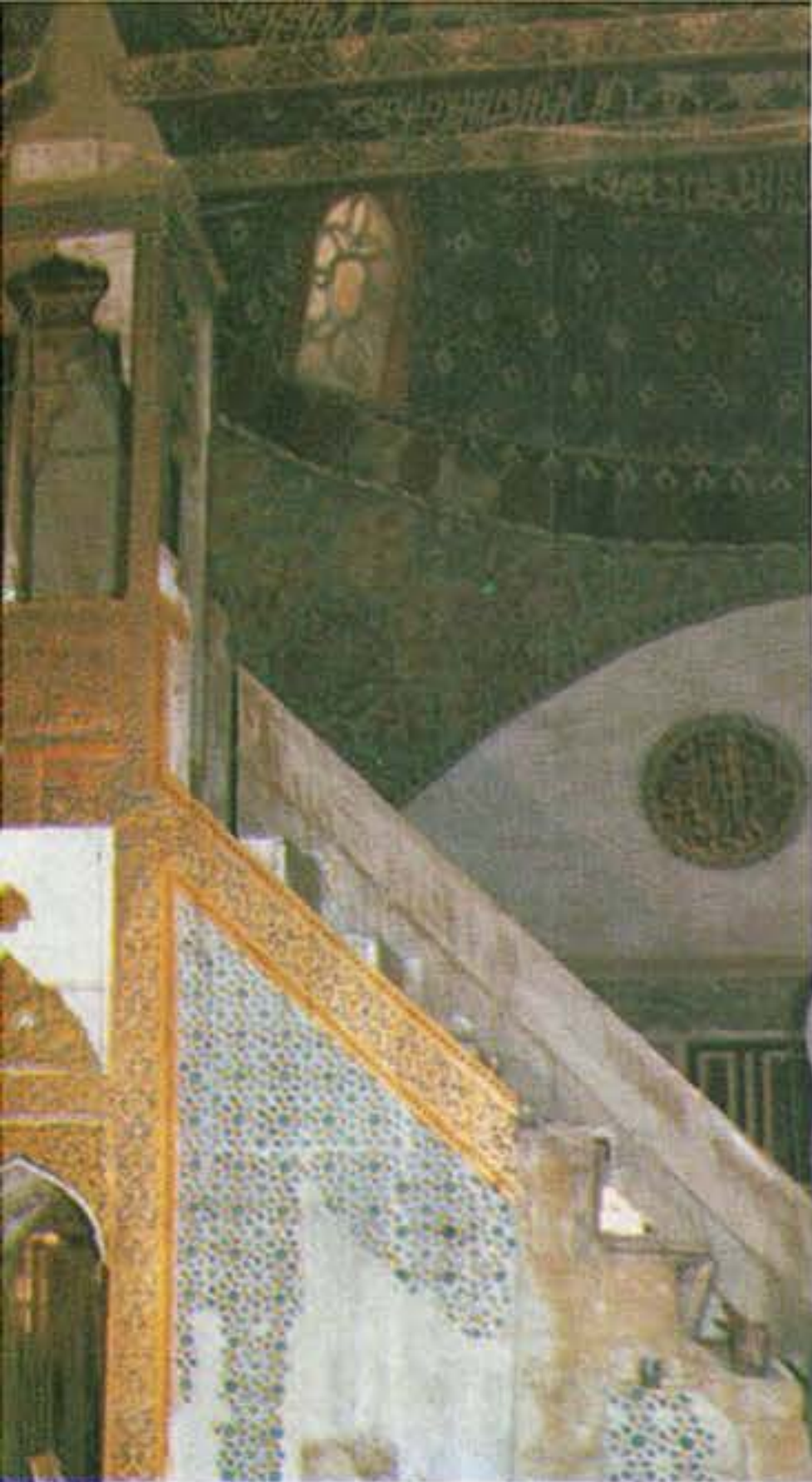
Minbar of Soliman Pasha Al-Khadem during restoration.
