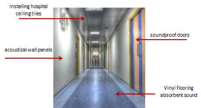
Fig. 15: Finishing materials for corridors inside the nursing unit so that they are soundproofed
