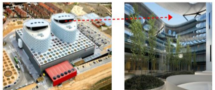
Fig. 5: The use of large surfaces of openings in Rey Juan Carlos Hospital, Móstoles, Madrid, Spain
