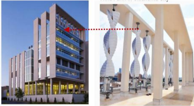
Fig. 10: (OklahomaMedical Research) ,VengerWindUnveils World’s Largest Rooftop Wind Farm in Oklahoma City http://www.405magazine.com/September-2012/
