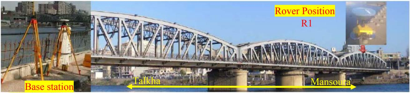
Figure 1. Mansoura Railway Bridge and GPS monitoring system
