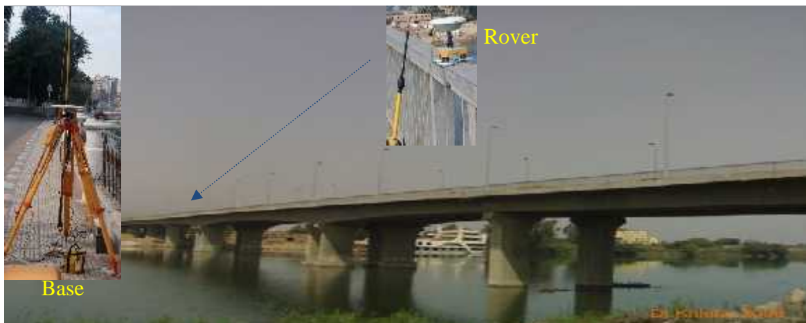
Figure 1: Mansoura Bridge and GPS monitoring system design
