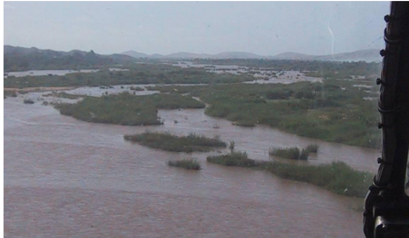
Photo 3: Flooded area along Coporolo River
