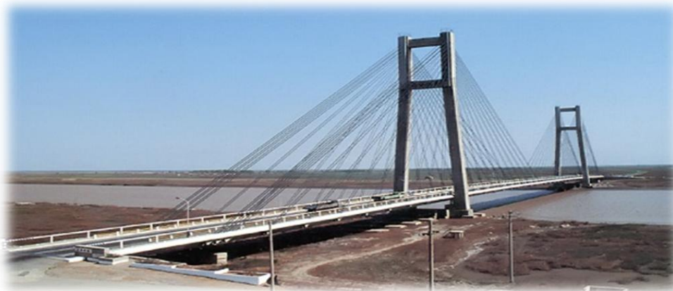
Figure 1 Yonghe Bridge southern tower general view
