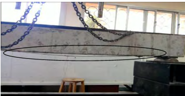
Figure 7 Failure and crack pattern of specimen (B3).
