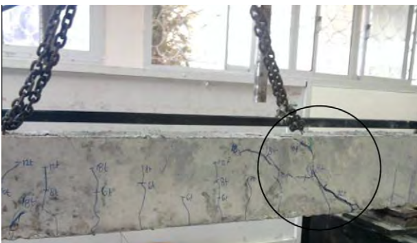
Figure 8 Shear failure and crack pattern of specimen (B4).
