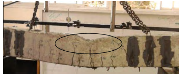
Figure 9 Failure and crack pattern of specimen (B5).
