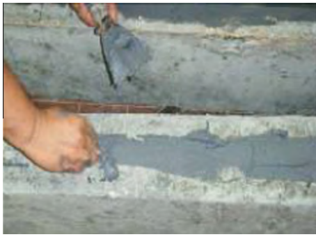
Figure 2 Applying the epoxy resin on the concrete surface.
