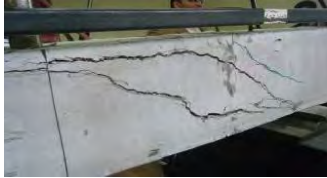
Figure 7 Crack patterns of control specimen
