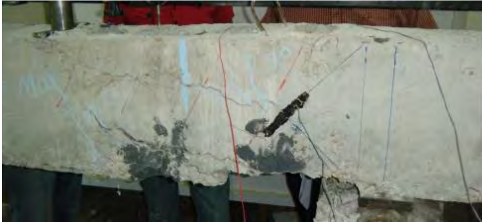
Figure 9 Crack patterns of specimen S-IER
