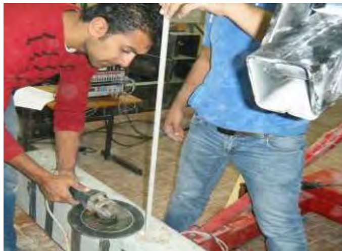
Figure 3 Installing of reinforcement in specimen IER
