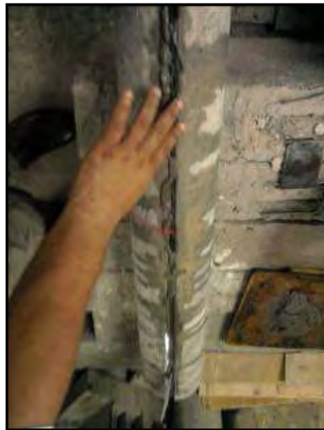
Figure (5) embedding the external reinforcement into the column concrete cover
