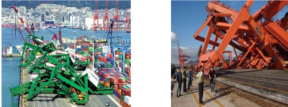
Fig. 1 Crane collapse by Typhoon in Pusan ports (Gamman, Jasungdae 2003)
