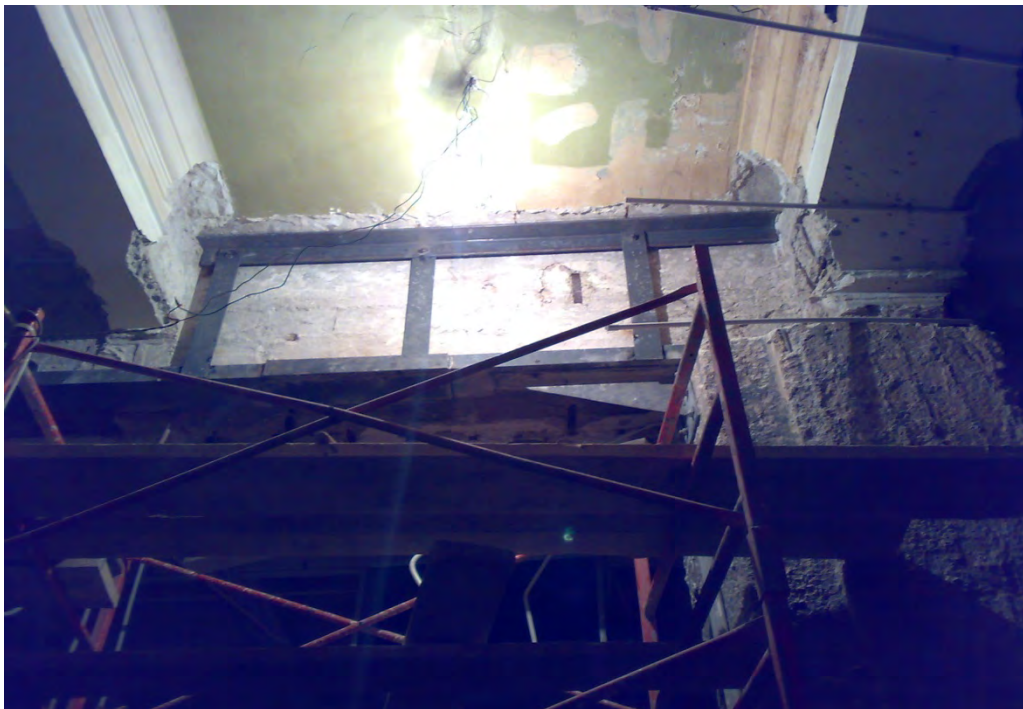
Figure C.11 Beam steel jacketing.
