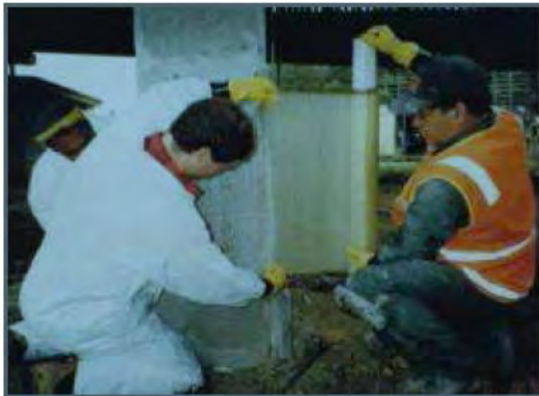
Wrapping with Glass Fiber
