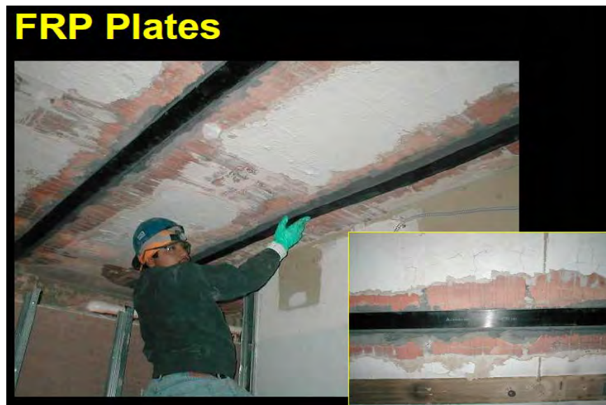
Figure 6.6 Strengthening of RC slab by using FRP.
