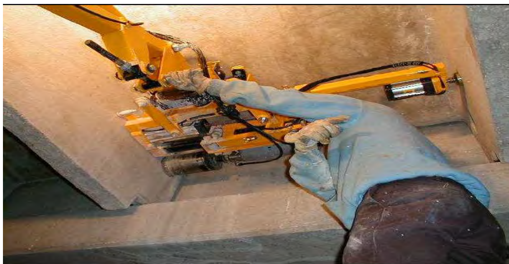
Figure 6.12 Cable jacking from life end.
