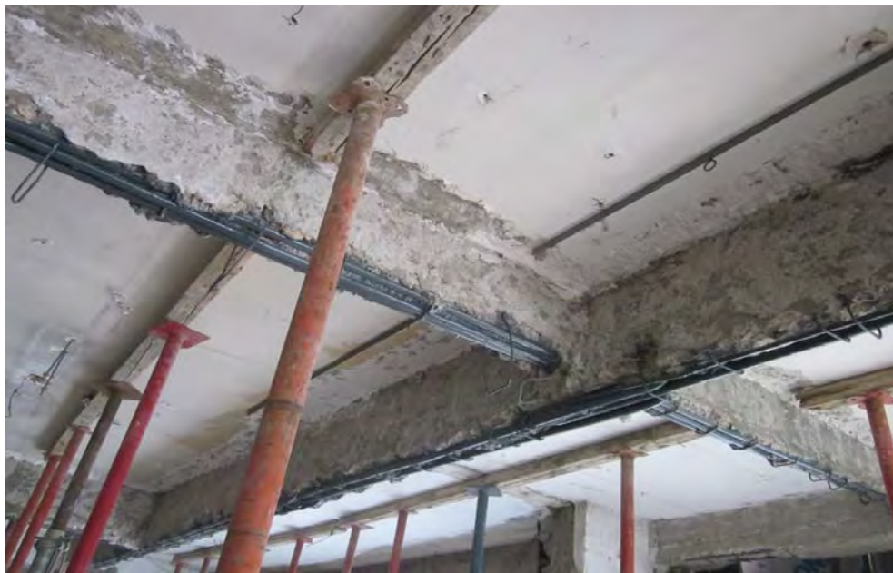
Figure B.8 Jacking process during cover removing.
