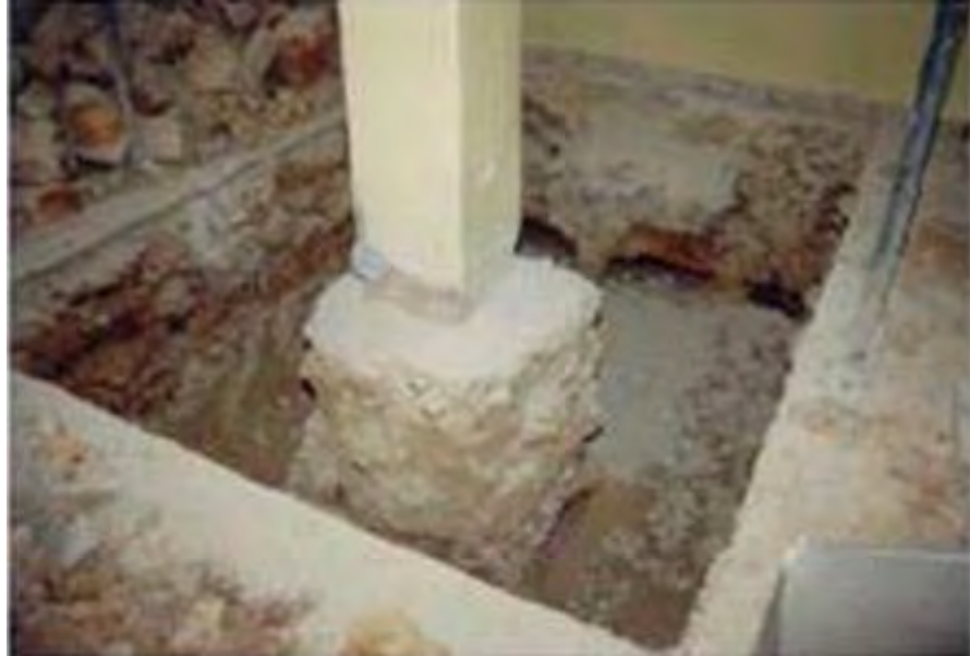
Figure 3.3 Excavation around the footing.
