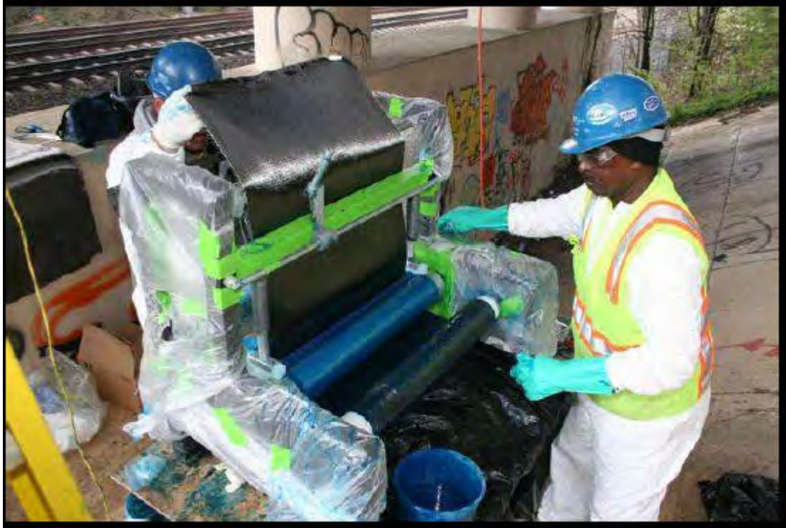
Figure 5.10 CFRP saturator.
