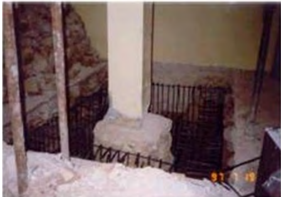
Figure 3.4 Harding the surface and installing the dowels
