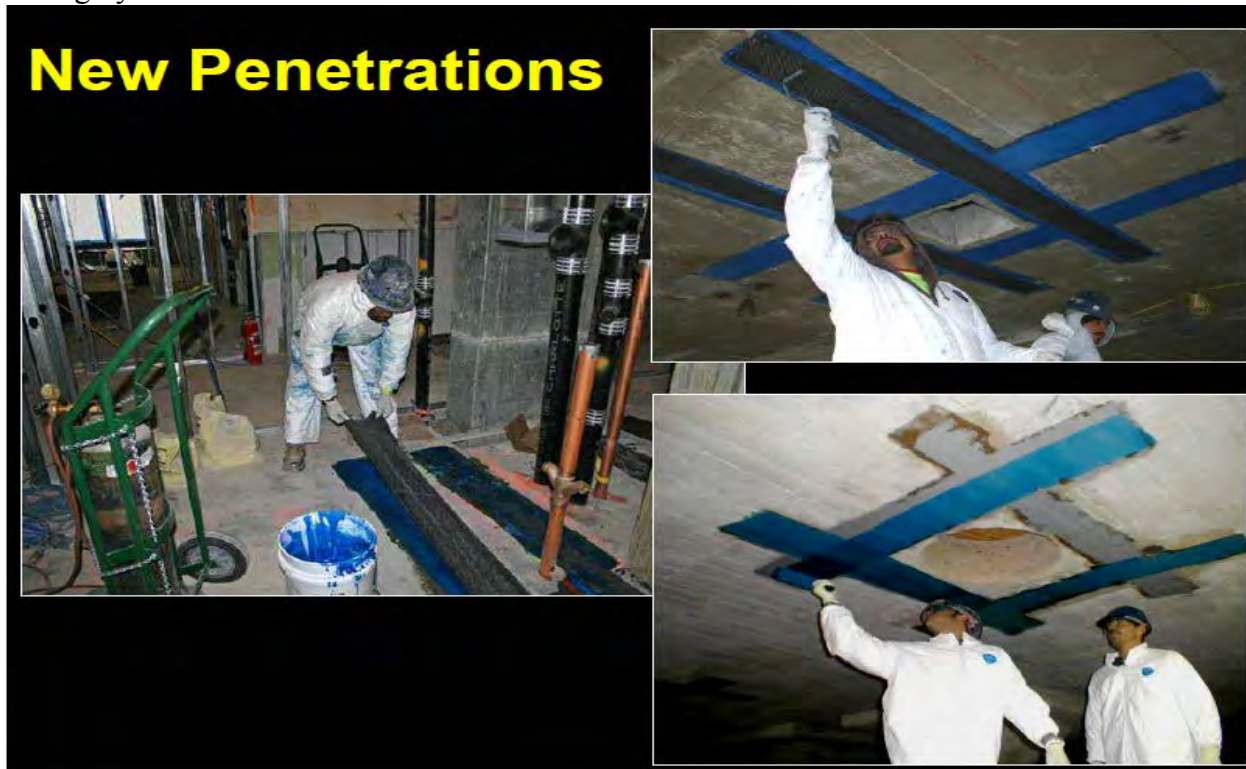
Figure 6.14 Installing a CFRP plates around the openings.
