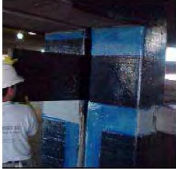
Wrapping with Carbon Fiber
