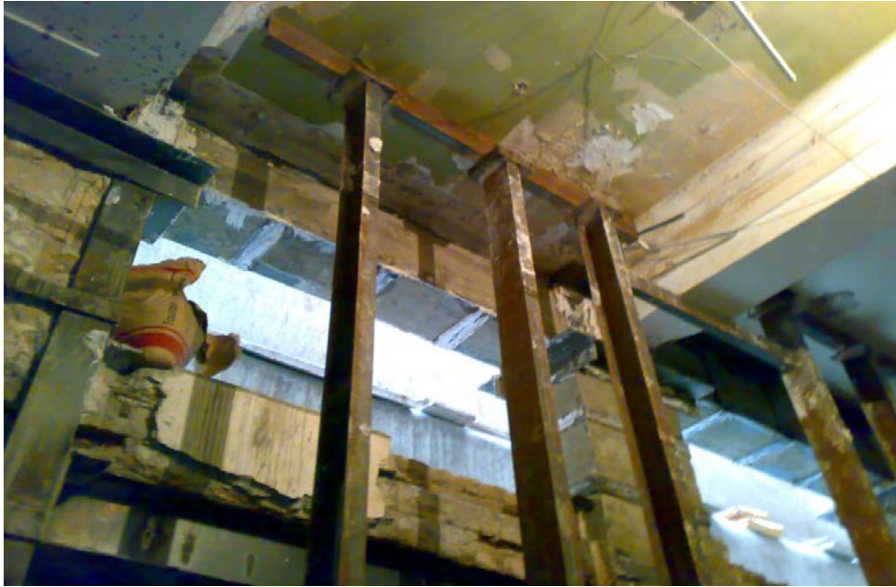
Figure C.16 Jacking process during column strengthening.
