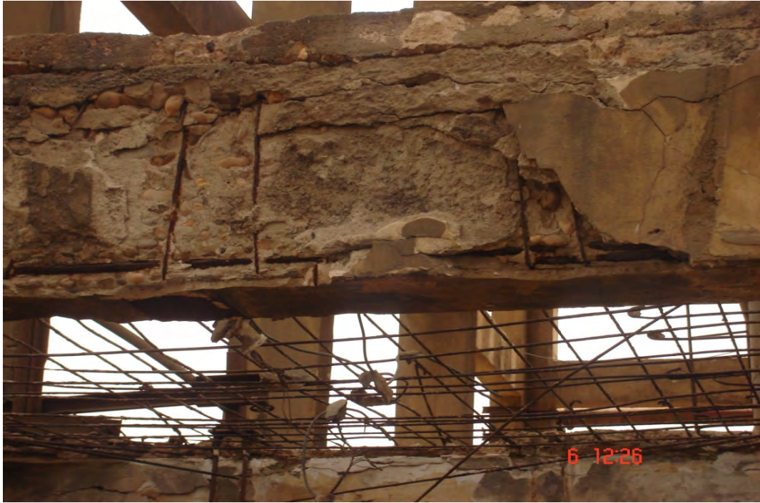
Figure A.34 Damaged Beam in the first level.
