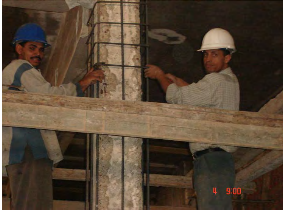
Figure A.12 Installing reinforcement steel jacket of the columns.
