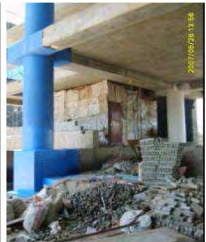
RC Columns after Completion of FRP Wrapping
