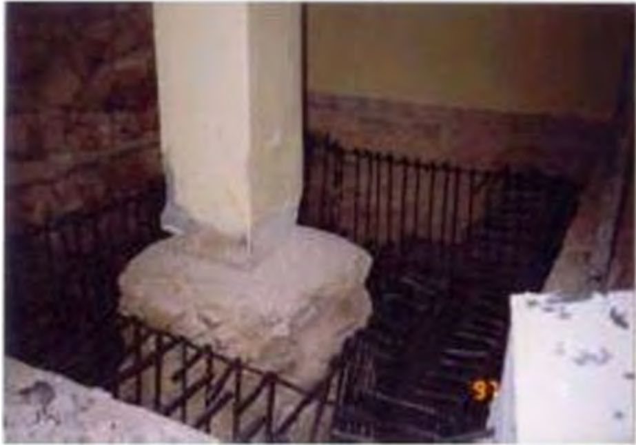
Figure 3.5 Installing the main steel.
