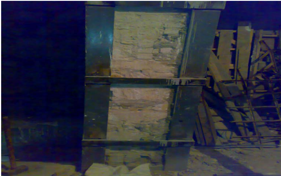
Figure C.15 Column steel jacking.
