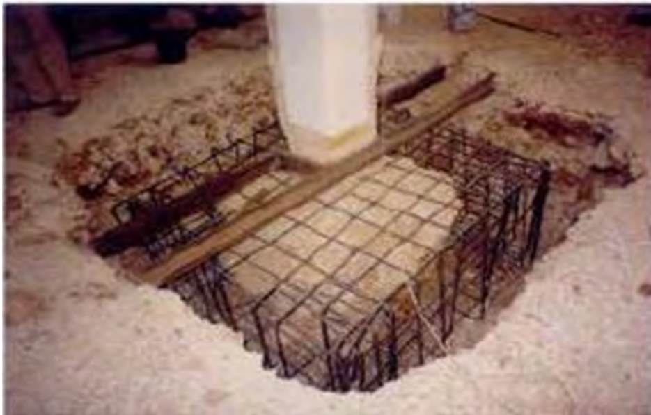
Figure 3.6 Completing the jacket.
