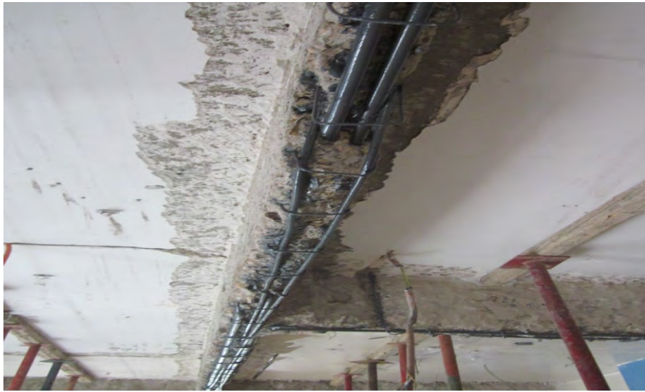
Figure B.7 Cover removing
