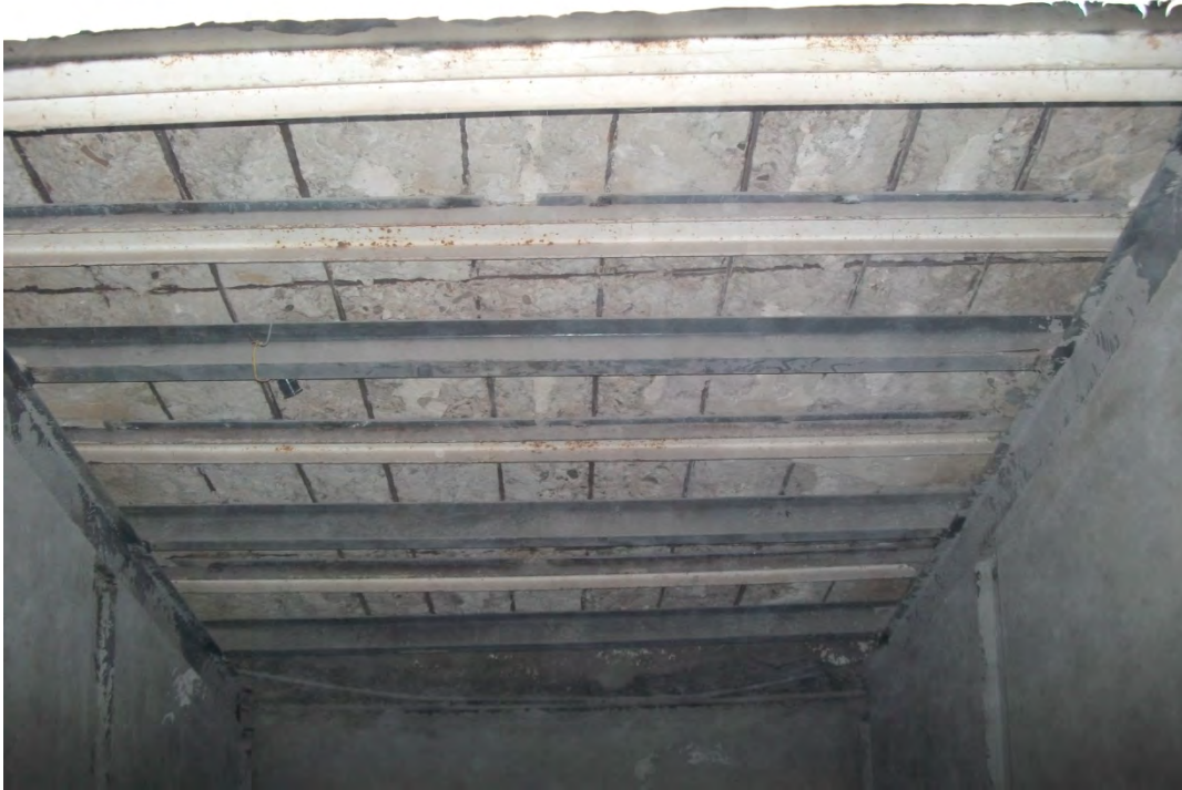
Figure C.10 Stair slab strengthened by steel beams.
