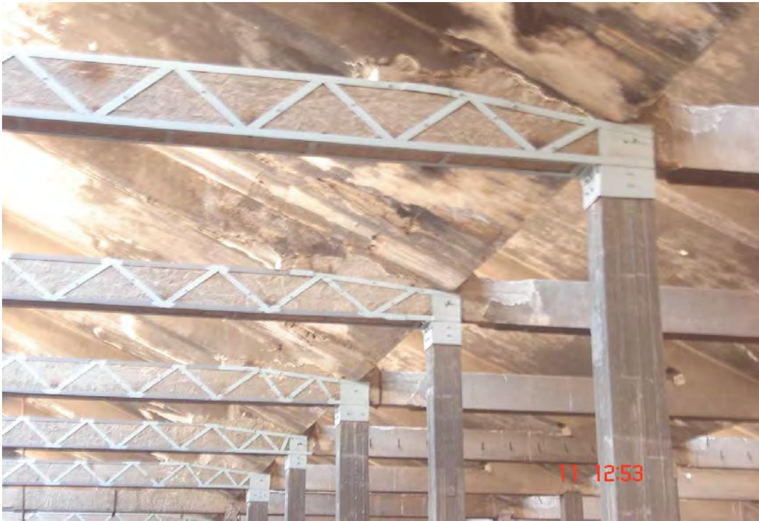
Figure A.28 Completing girders strengthening.
