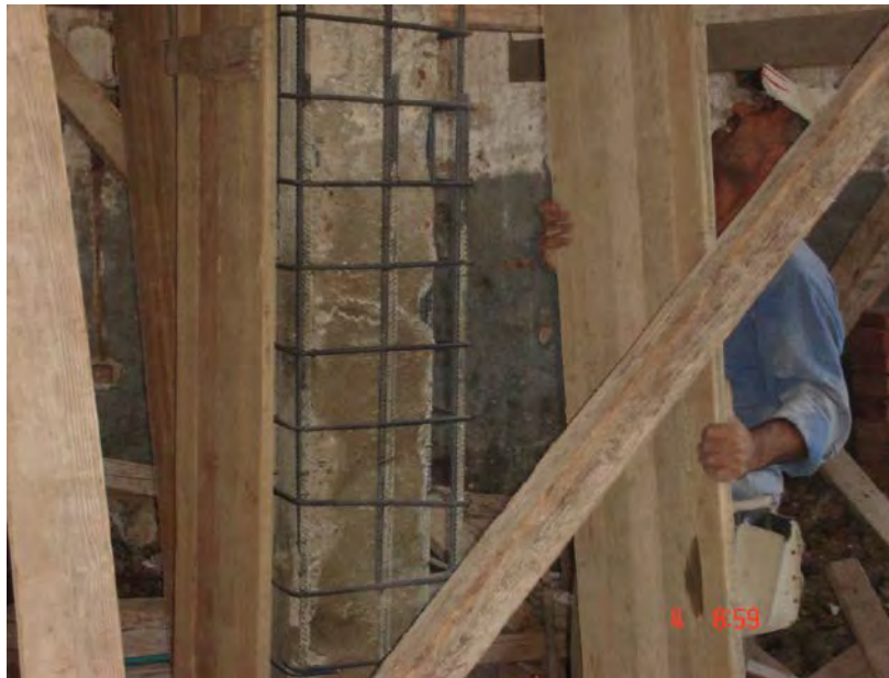
Figure A.15 Preparing casting of the concrete jacket.
