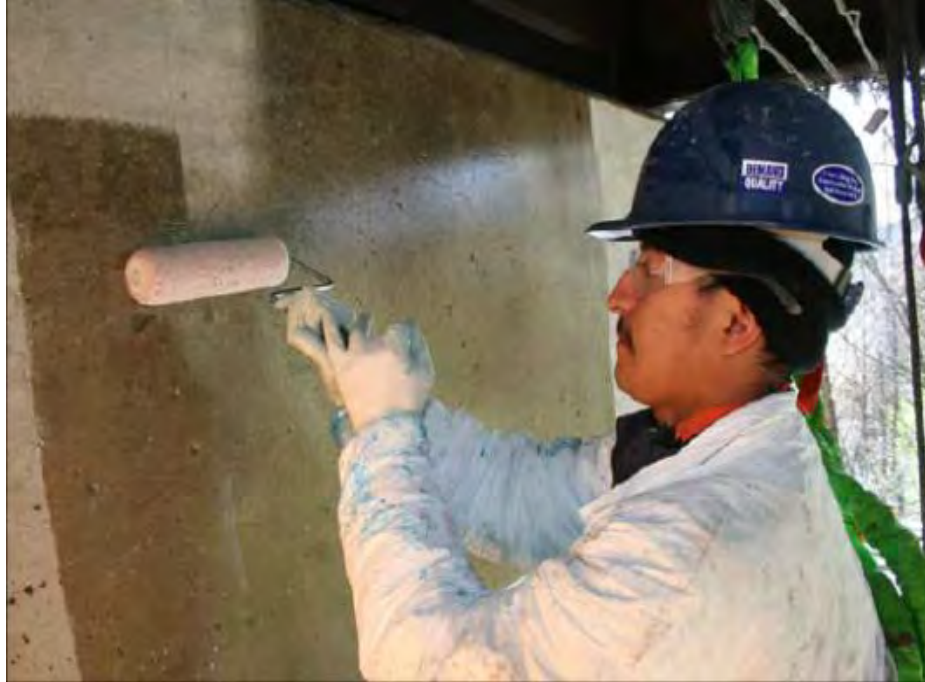
Figure 5.8 Application of primer .
