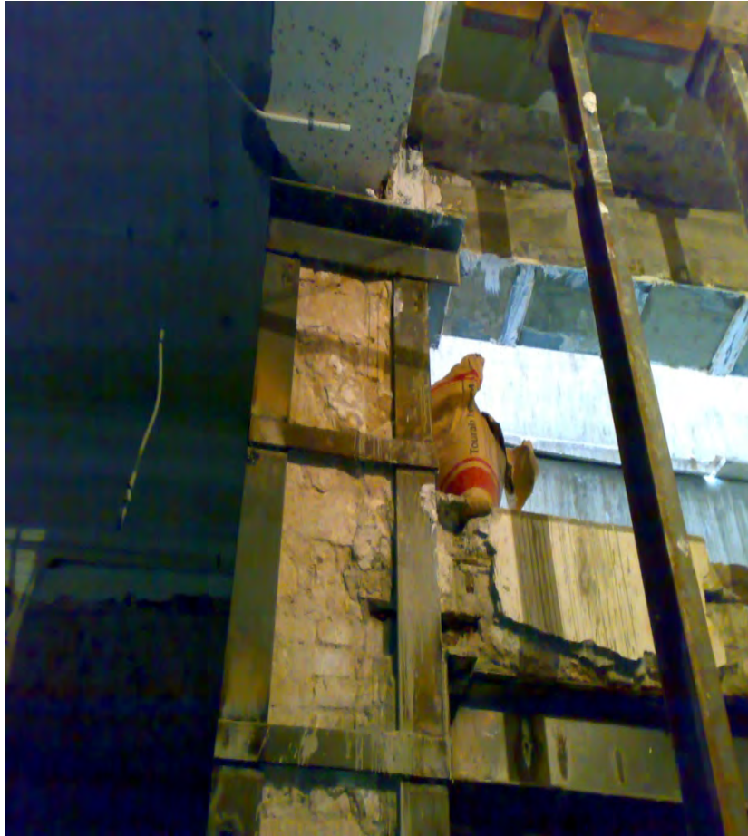
Figure C.18 Steel jacket connection with slab.
