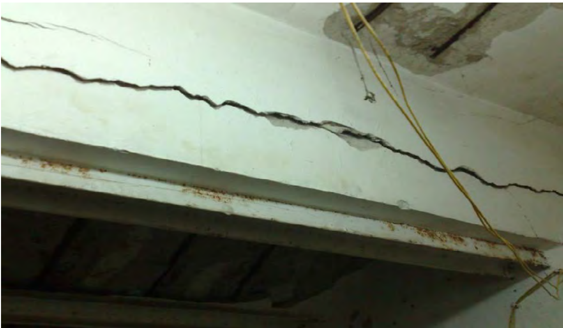
Figure C.4 Damaged beam.
