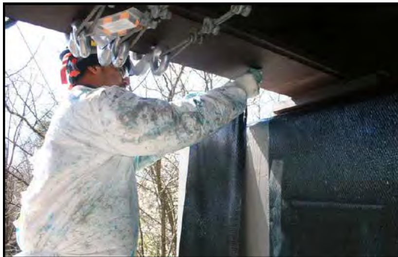
Figure 5.11 Fiber lay up.
