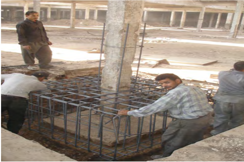
Figure A.8 Installing the main steel of the footing jacket.
