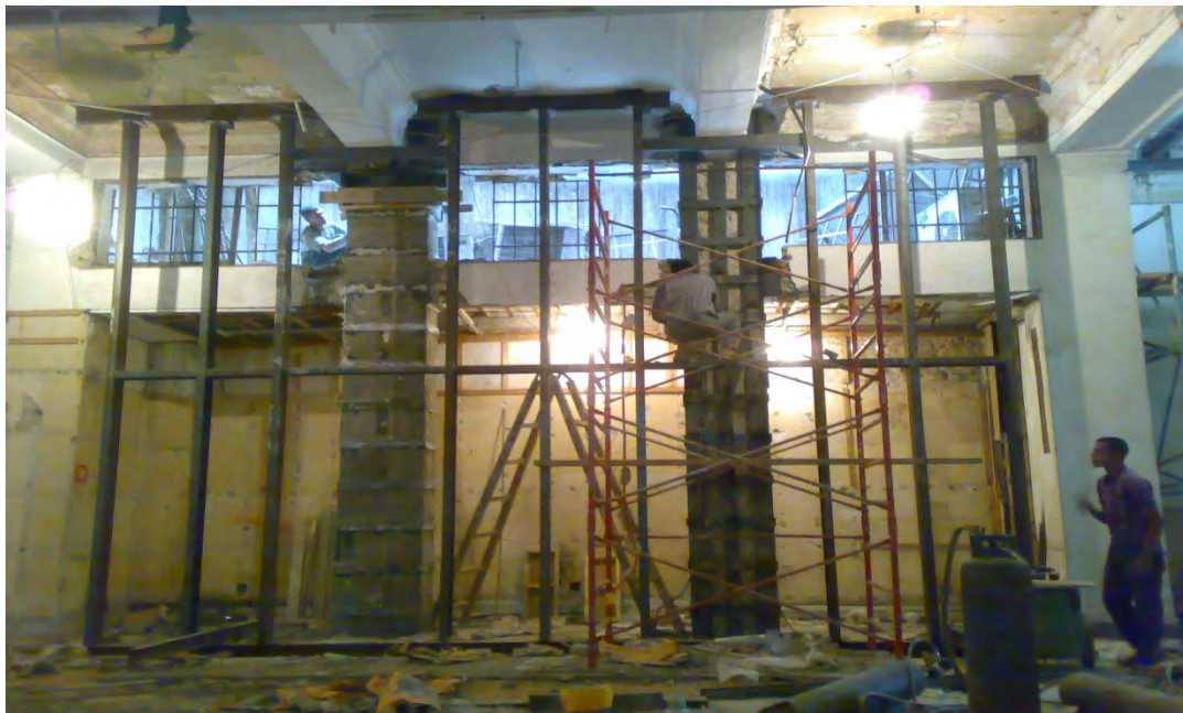
Figure C.17 Completing column steel jacketing.
