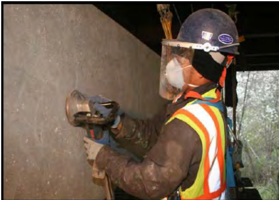
Figure 5.7. Grinding to the surface.
