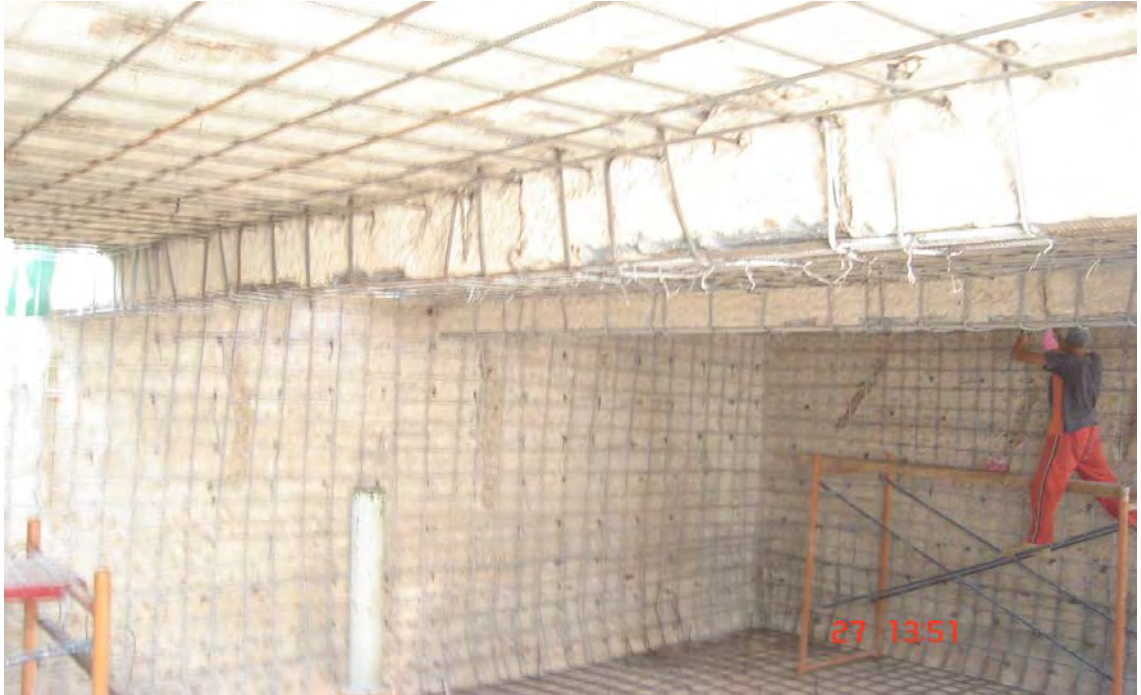
Figure A.41 Installing a new reinforcement mesh.
