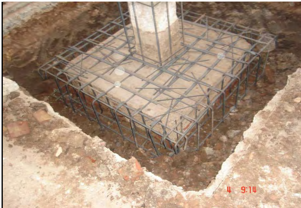
Figure A.9 Completing the main steel of the footing jacket.
