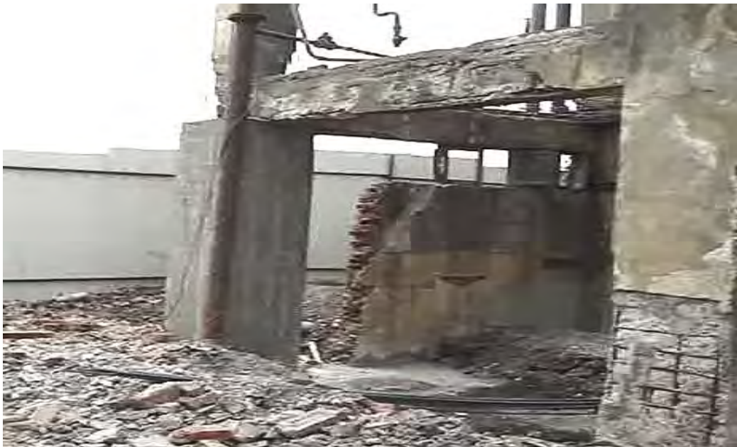
Figure A.34 Damaged Beam in the first level.
