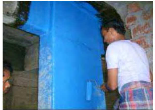
Application of Saturant on FRP Wrapping
