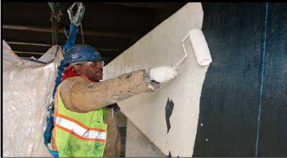
Figure 5.14 Topcoat installation .
