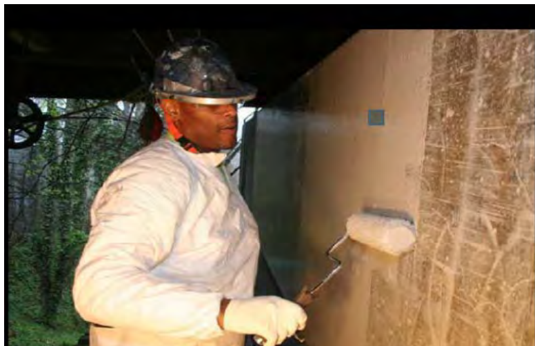
Figure 5.9 Application of saturant.
