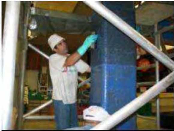
Application of Saturant on FRP Wrapping
