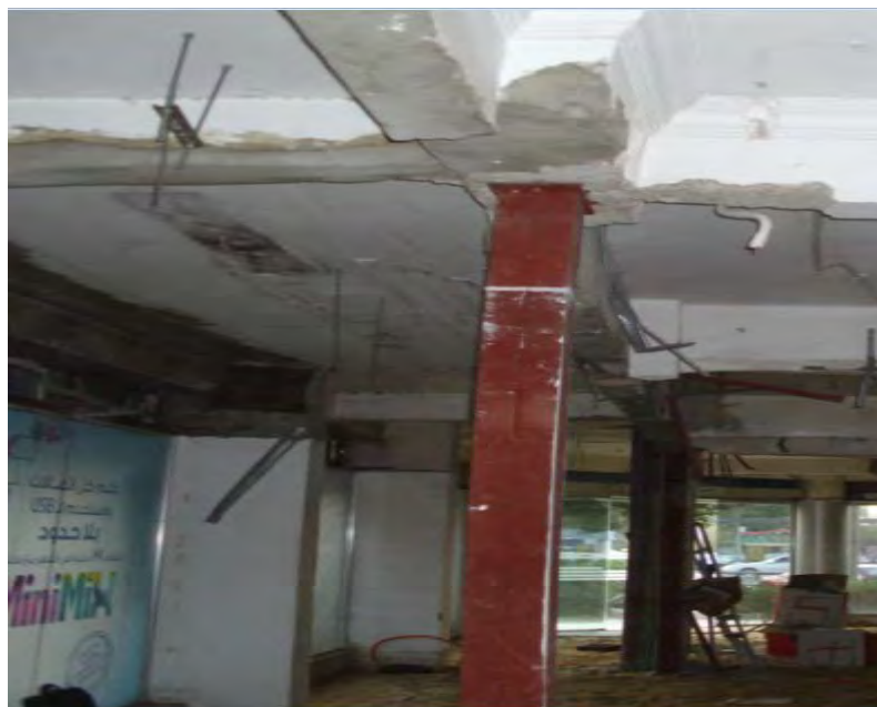
Figure B.6 RC Column removed by a steel column.
