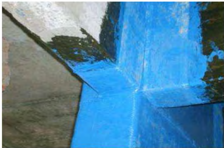
RC Columns after Completion of FRP Wrapping
