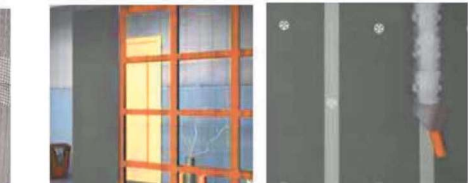
Fig.20. The Installation on Timber Working
