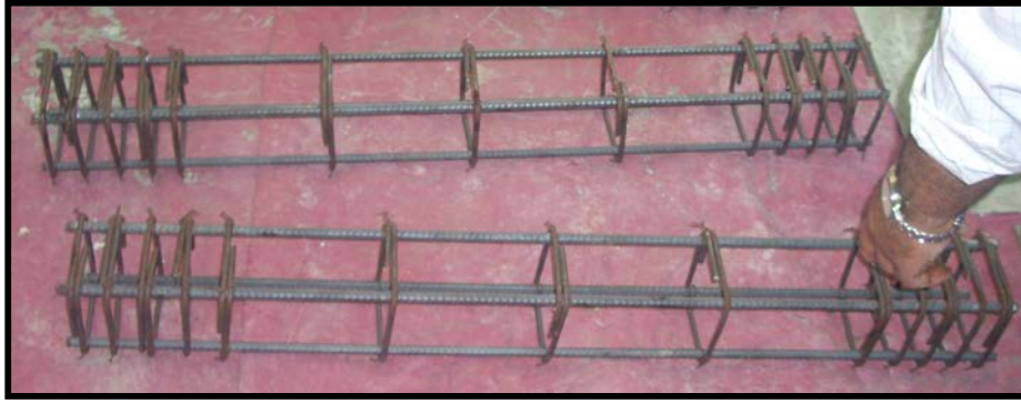
Fig. 3.7 Reinforcing steel cage
