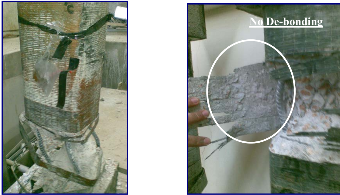
Fig. 4.6 Failure in Columns C.F.-200-4, and R.W.-200-8
