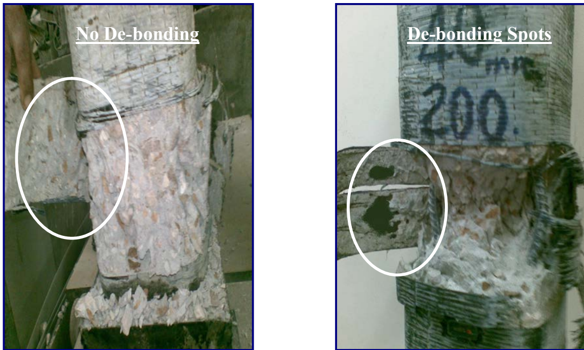
Fig. 4.7 Failure in Columns S-200-12, and G-200-24
