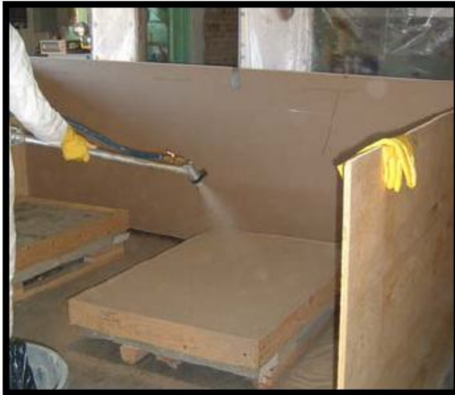
Fig.2.11 Slab Strengthening and Insulation details and spray application
