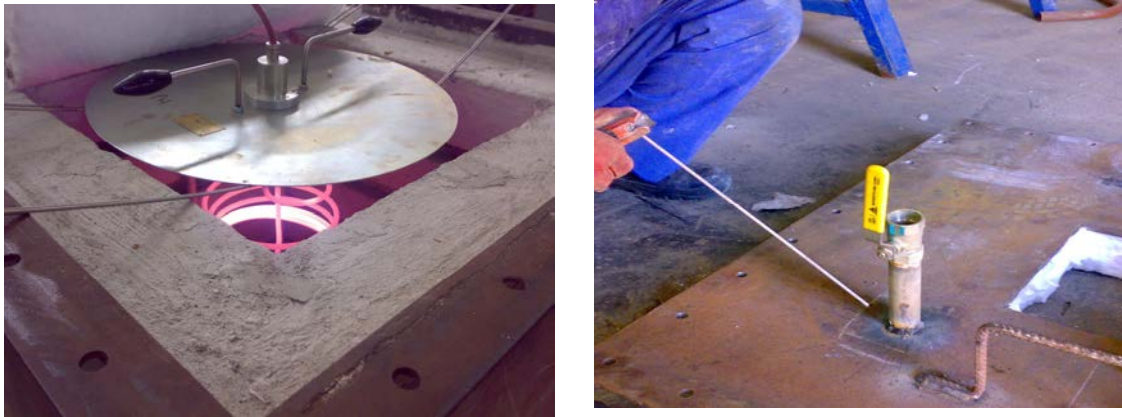
Fig. 3.14 Furnace curing and nozzle welding
