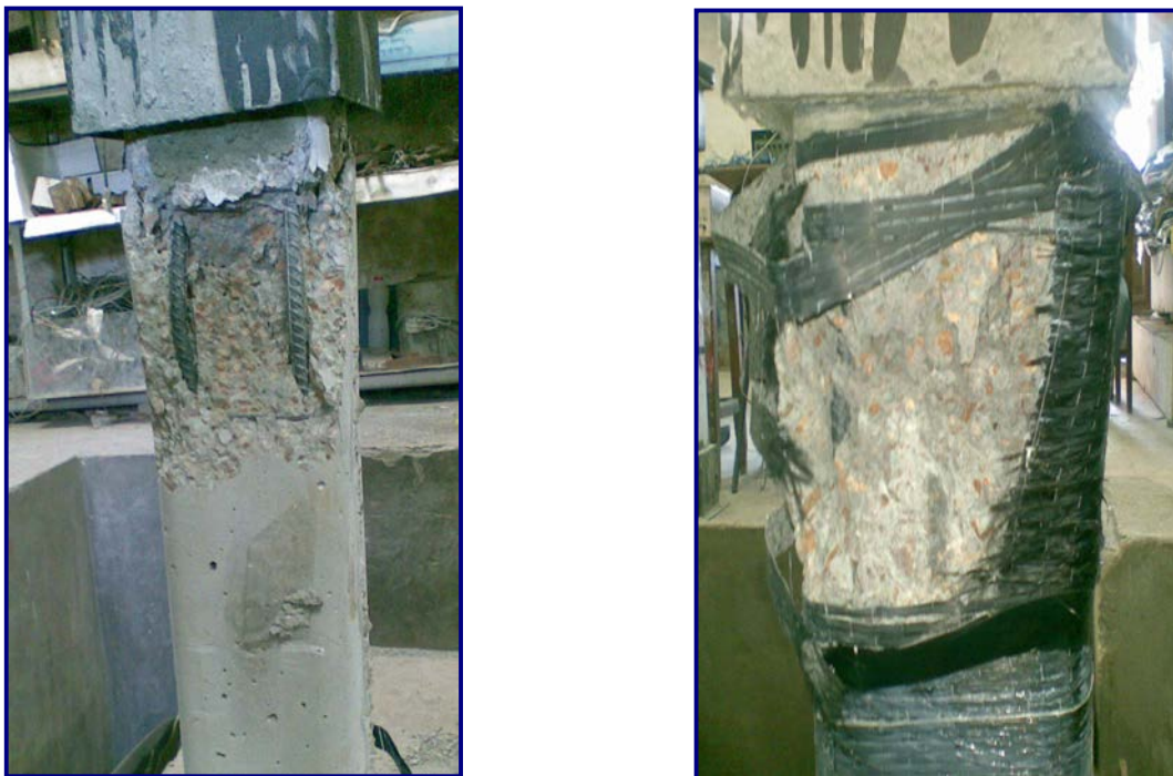
Fig. 4.1 Failure mode for both confined and un-confined columns at room temperature
