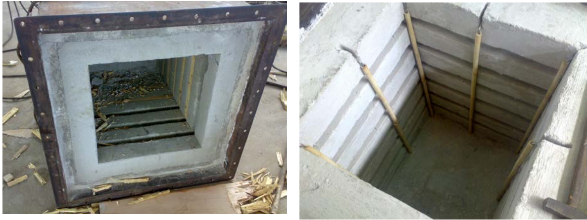
Fig. 3.11 Grooving the coils shelves and installing the coils hinders
