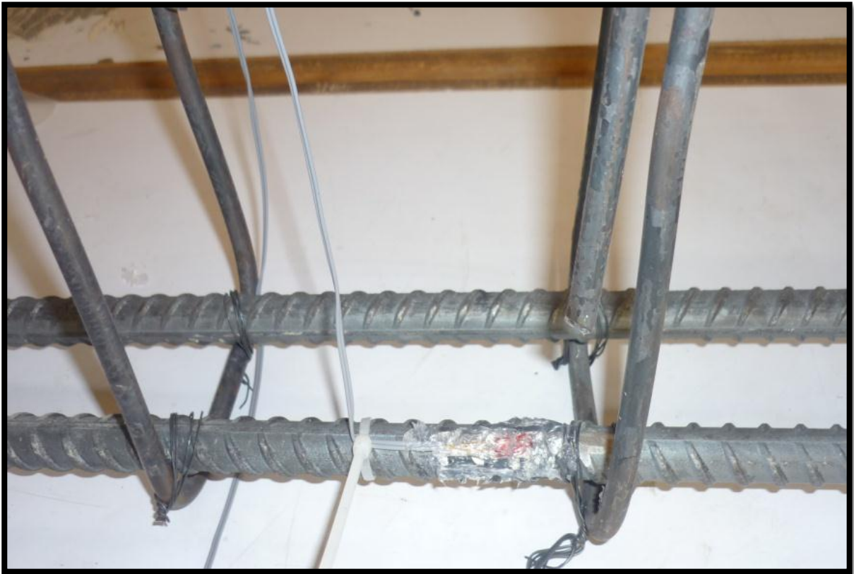
Fig (3.6). Strain Gage at Mid-Span of Beam
