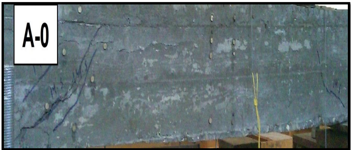
Figure (4.1) Crack Patterns for specimen (A-0).
