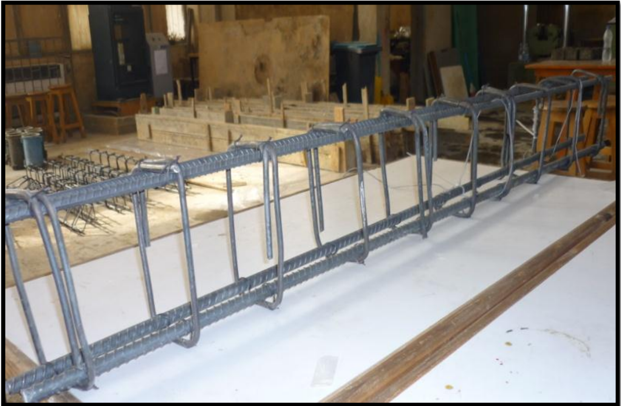
Fig (3.4). Reinforcement Details of Beam
