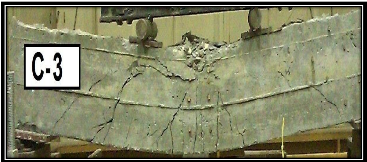
Fig (4.34). Crack Patterns for specimen (C-3).
